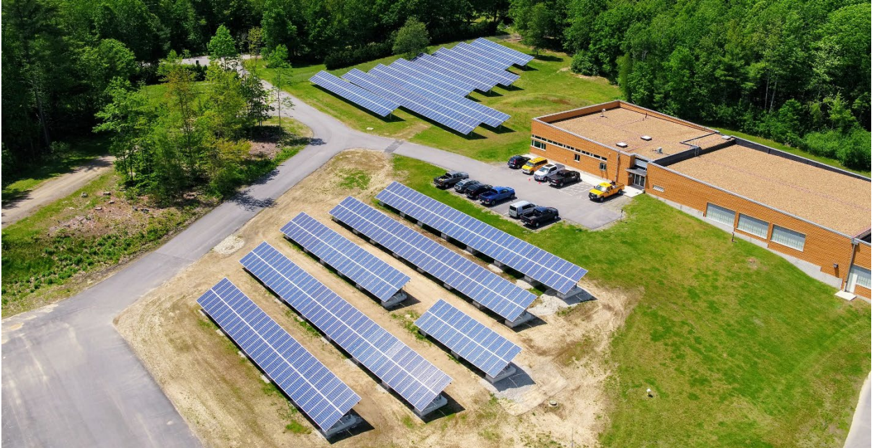
Solar Photovoltaic (PV) Array at the Madbury Water Treatment Plant
