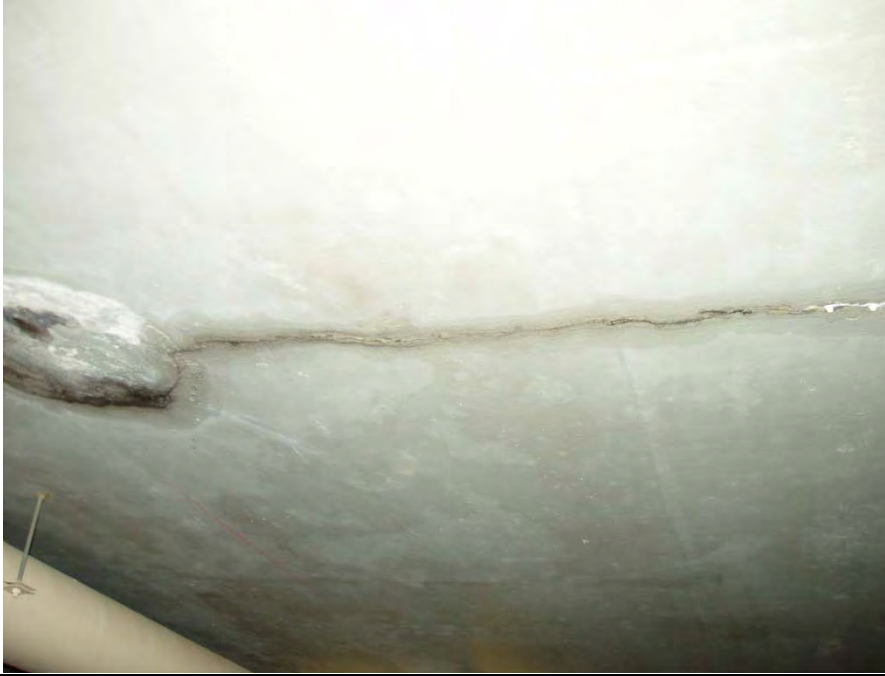
Photo 5: Mudwell Gallery Leaking Cast in Place Concrete Roof Surface.
