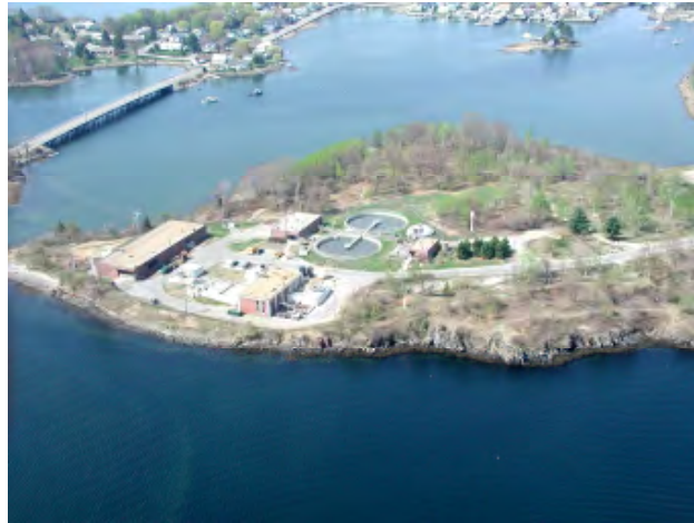
Figure 1-2. Peirce Island WWTF Aerial View
