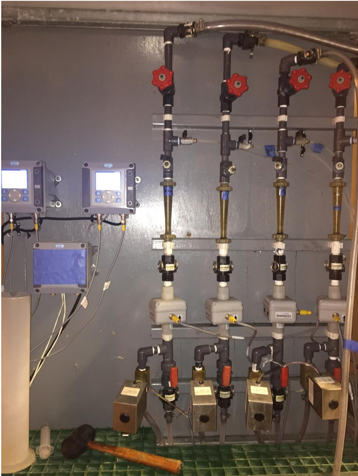
In-stream flow and turbidity meters, and computer-control units for Combined Raw water (left), Filter 1 effluent (second from left), and Filter 2 effluent (second from right).
