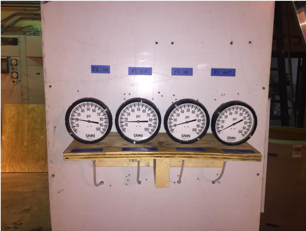
Pressure gauges to monitor influent and effluent pressures for each filter.
