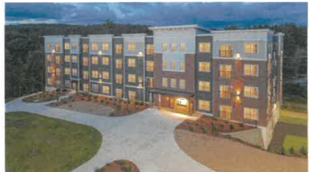
4-STORY RESIDENTIAL BUILDING W/ MULTIPLE MATERIALS AND COLORS
