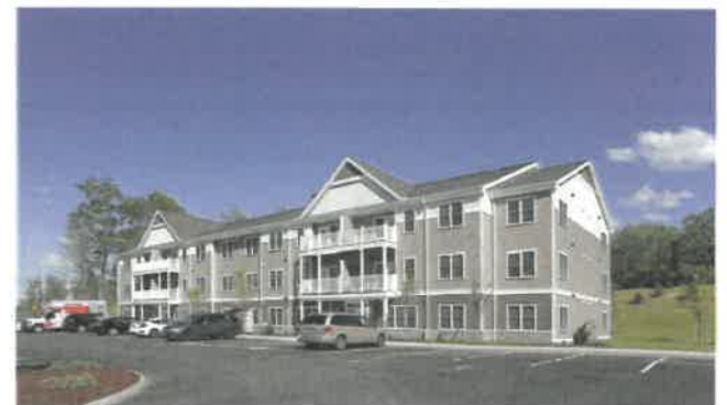
5-STORY SMALL RESIDENTIAL BUILDING
