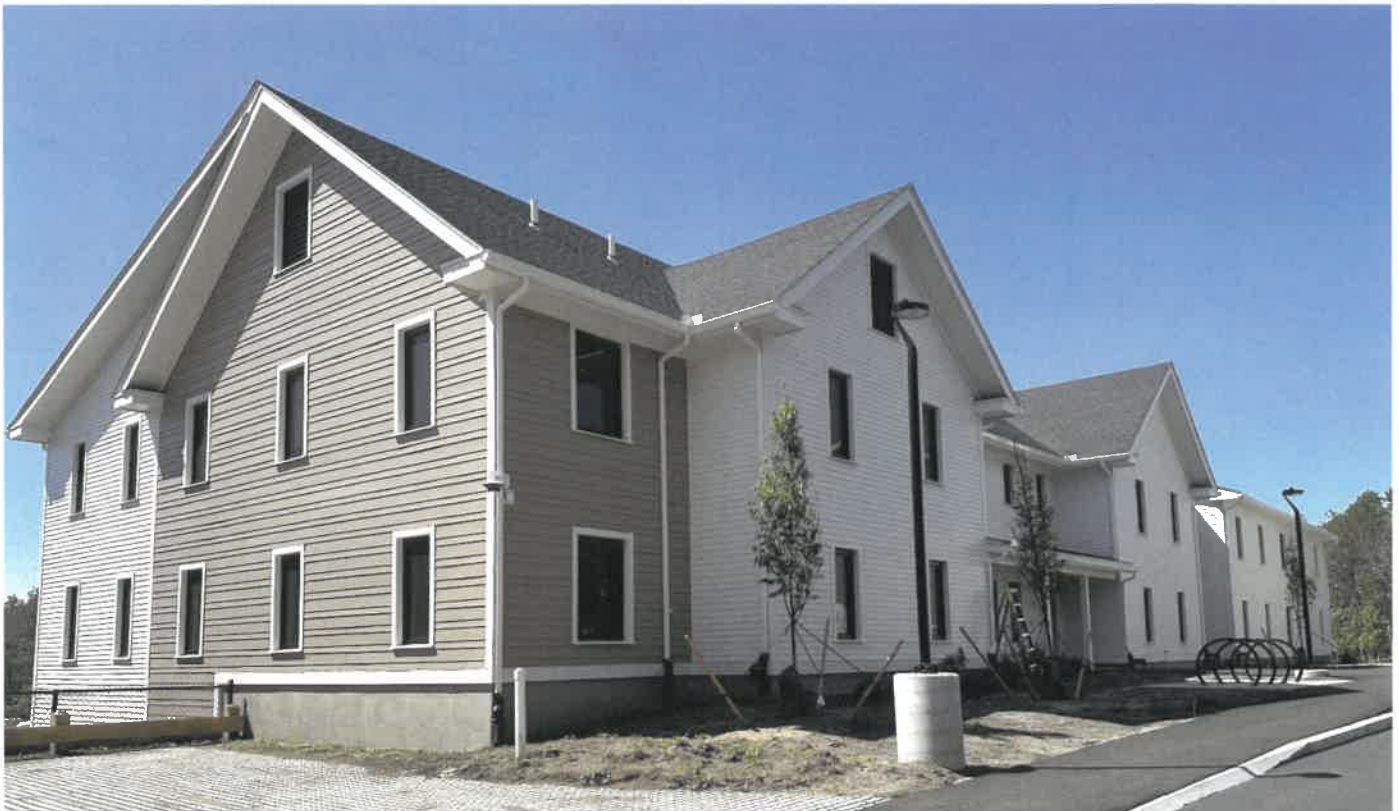
LeClair Village in Mashpee on Cape Cod. Construction is expected to complete later this summer.
