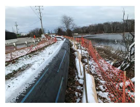
Photo 3: Construction Fencing Along the Length of Temporary Sewer Force Main
