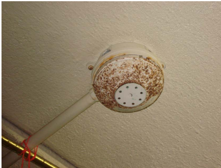
Photo 7: Filter Building Smoke Detector Corrosion
