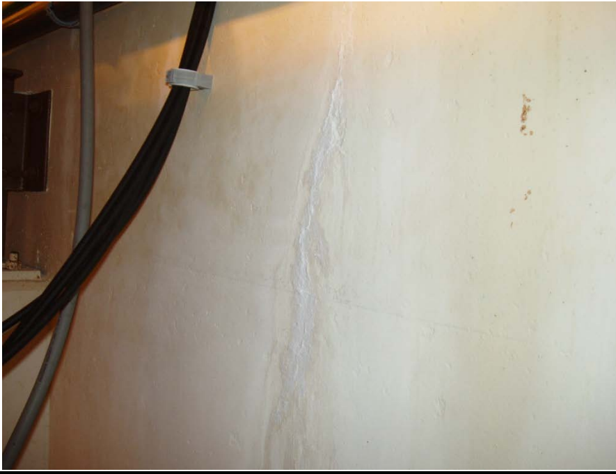
Photo 7: Clearwell Gallery Wall Surface with Efflorescence.
