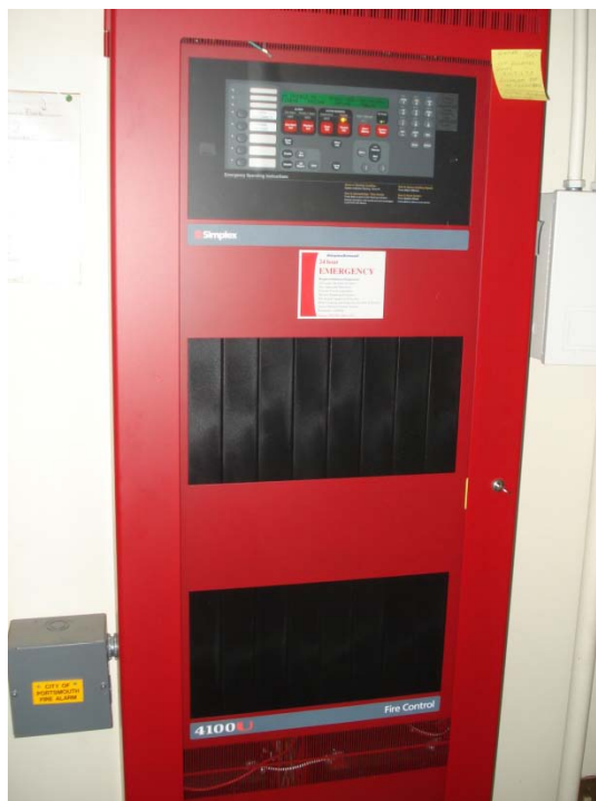
Photo 5: Control Building Main Fire Alarm Panel
