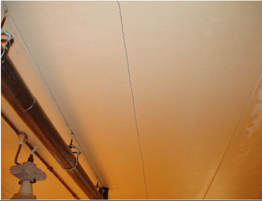
Photo 11: Filter Room Precast Hollow Core Concrete Roof Plank Crack.
