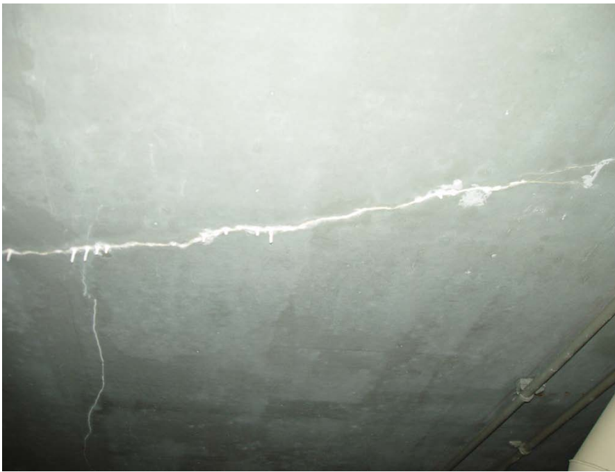
Photo 4: Mudwell Gallery Non-leaking Cast in Place Concrete Roof Surface.
