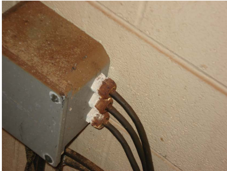
Photo 6: Filter Building Raceway Corrosion
