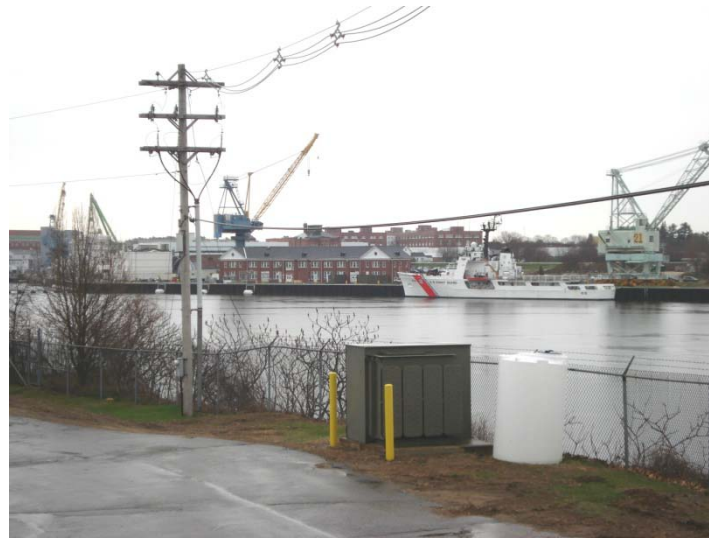
Photo 1: Utility Riser Pole and Transformer
