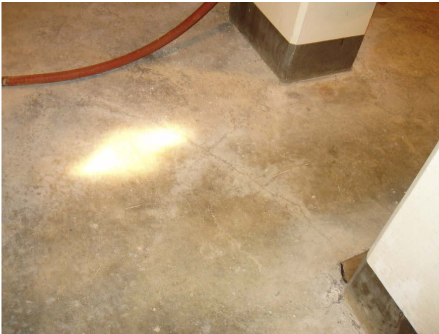
Photo 8: Clearwell Gallery Spider Cracks in Floor Surface.
