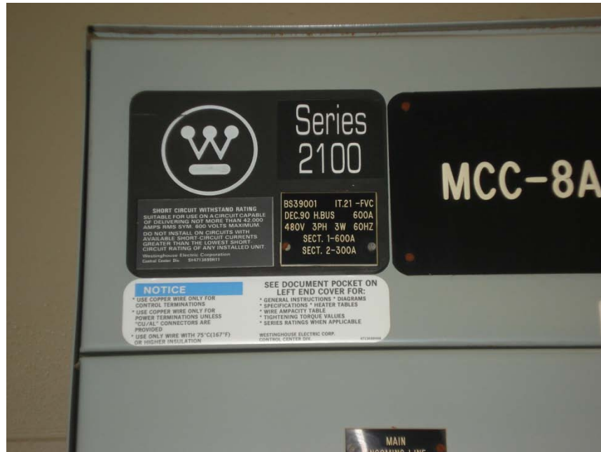
Photo 3: Motor Control Center Data Nameplate
