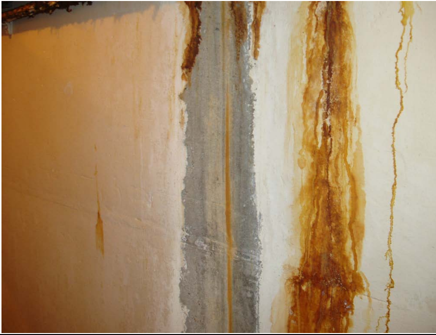
Photo 9: Clearwell Gallery Wall Surface with Chemical Corrosion.
