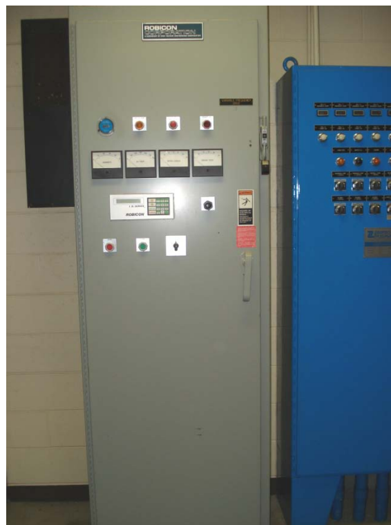
Photo 4: Robicon VFD for Effluent Pumps
