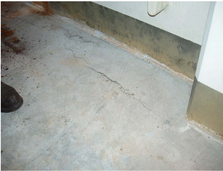
Photo 6: Clearwell Gallery Delaminated Floor Surface.
