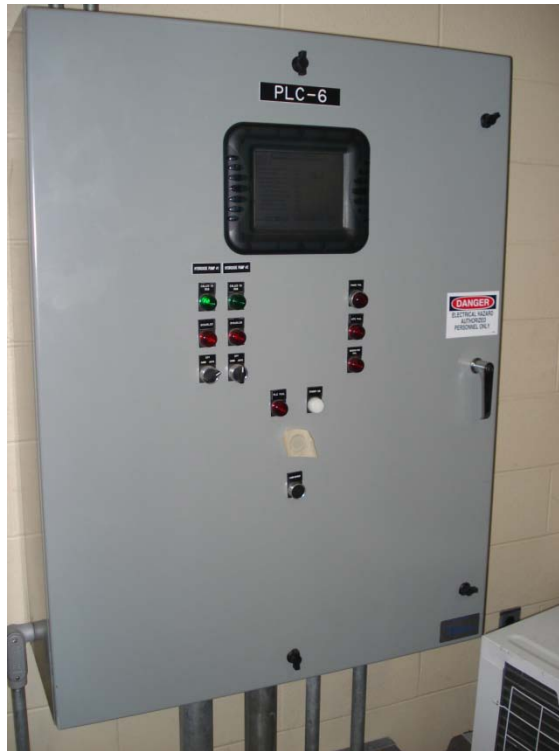
Photo 4: Filter Building SCADA System Panel
