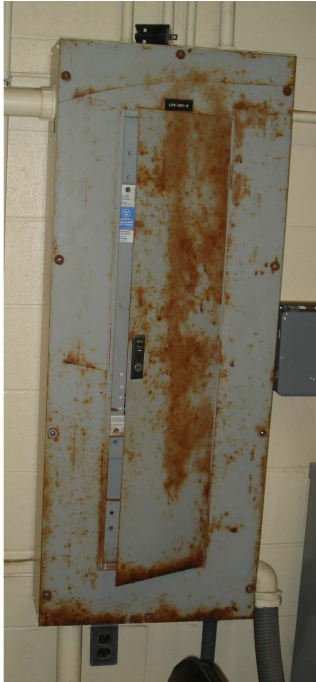
Photo 8: Filter Building Lighting Panel Corrosion
