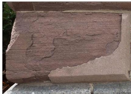
*Brownstone is very soft and susceptible to moisture damage. The surface of the brownstone has delaminated, the corner has spalled and a cementitious patch on the lower right corner is failing.*
