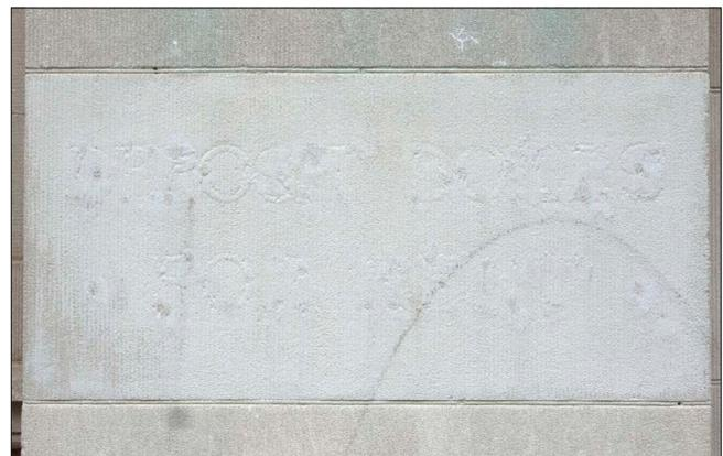
*It appears that an aggressive treatment was used to clean the limestone surface, resulting in a “bleached” effect when compared to adjacent stones. Although it is preferable to clean an entire wall surface, if spot cleaning is being considered, it is preferable to clean entire stone units ending at mortar joints as shown.*
