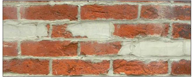
*Stucco patches are an inappropriate replacement for missing or damaged bricks. Missing or deteriorated brick should be replaced with units of the same dimension, appearance, texture and hardness as adjacent brick.*
