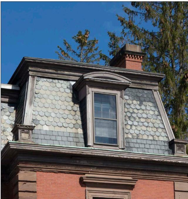
*This Mansard roof includes a combination of fishscale and rectangular slates. It appears that the lower rows of slate have been replaced, likely as part of a repair of the gutter flashing below the dormer window. (The decorative balustrade has been removed.)*
