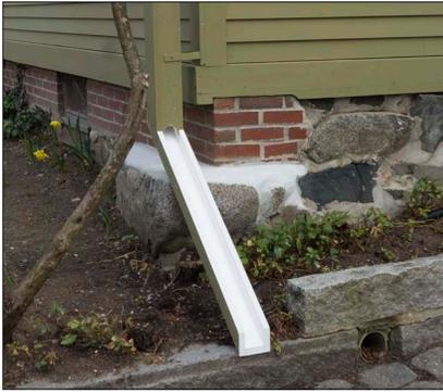
Downspouts direct storm water down the face of a building towards the ground. This example is encased in wood and includes an extension that discharges onto the driveway away from the foundation.
