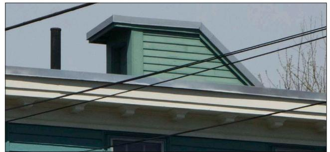
*This penthouse houses a stair to provide access to the roof, with the size minimized by the sloped roof form. The penthouse is held away from the roof edge, minimizing its visibility from the public way.*
