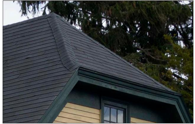
*Three-tab asphalt shingles, as seen on this jerkin-head roof, are a relatively inexpensive roof material, but will require more frequent replacement than other materials.*
