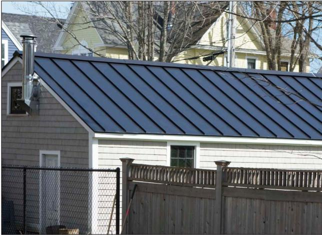
*Standing seam metal roofing installations have a distinct pattern of regularly-spaced ribs, which result in regular shadow lines.*
