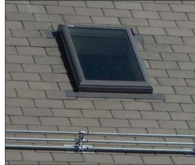
The skylight is installed at a rear elevation and is parallel to and only few inches above the roof surface. The glass and frame color are similar to the roof material, minimizing its visibility. Also note the snow guard.
