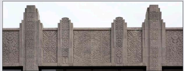
**Cornice:** The projecting horizontal moldings toward the top of the building wall at the roof edge.
