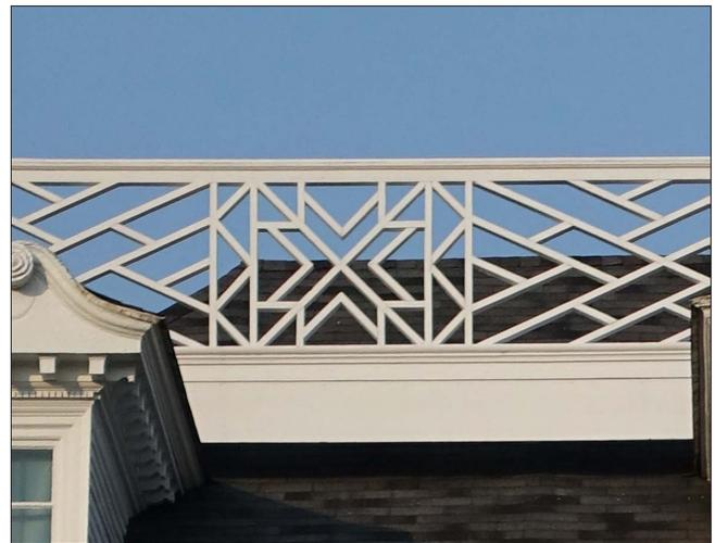
A widow's walk or roof railing is generally located where there is a change in roof slope.
