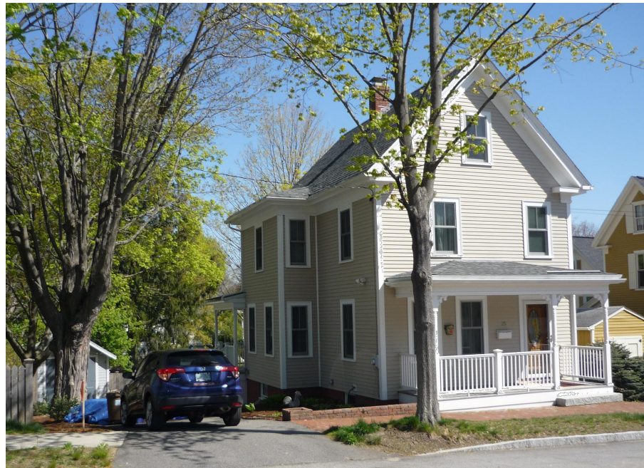
25 HAWTHORNE STREET – ON RIGHT SIDE / REAR
