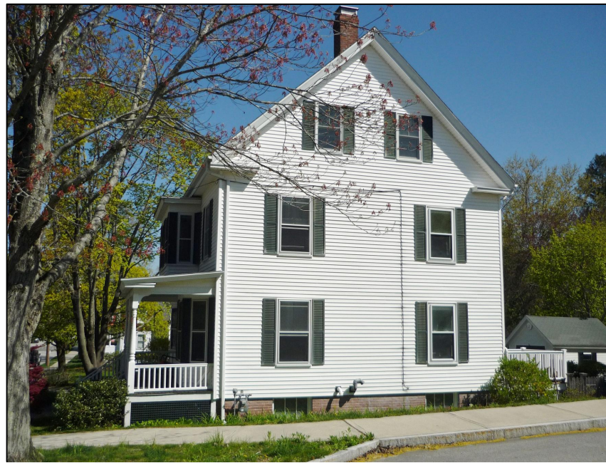
EXISTING HOUSE RIGHT SIDE (LEFT SIDE SIMILAR)
