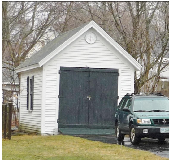
EXISTING SHED FRONT & LEFT
