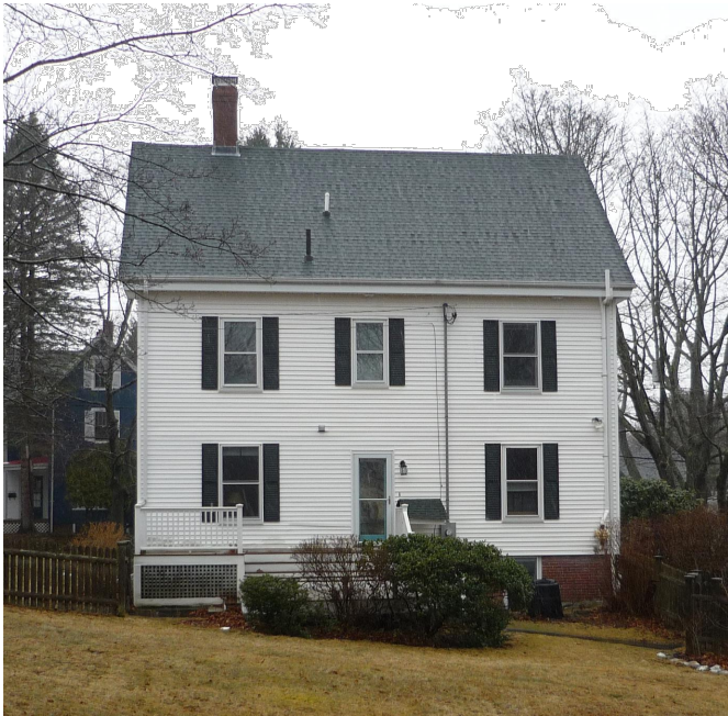
EXISTING HOUSE REAR
