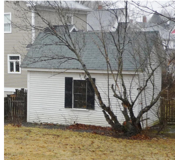
EXISTING SHED RIGHT SIDE & REAR
