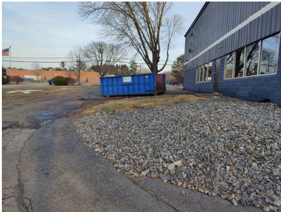
View of building looking to the east
