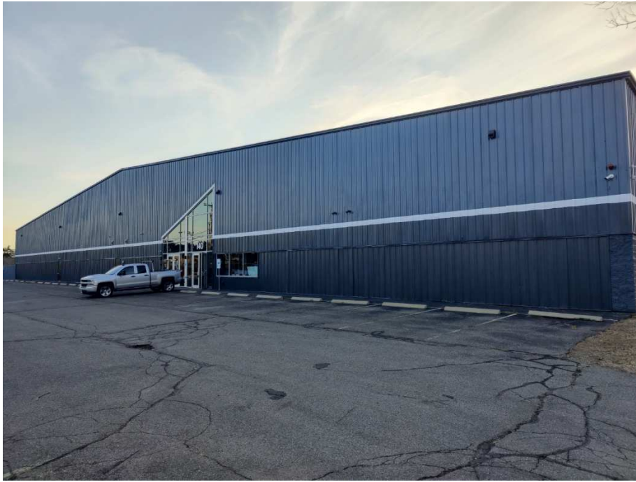
View of building looking to the west
