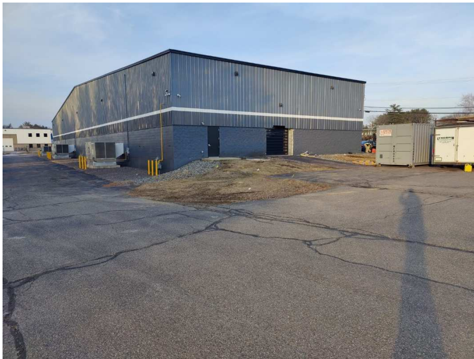
View of building looking to the east
