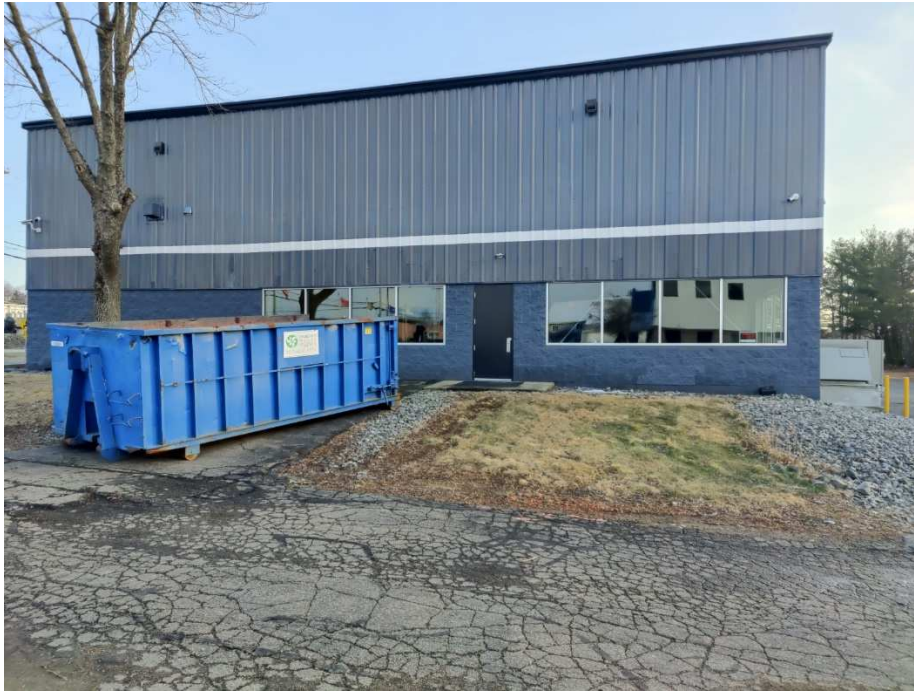
View of building looking to the south
