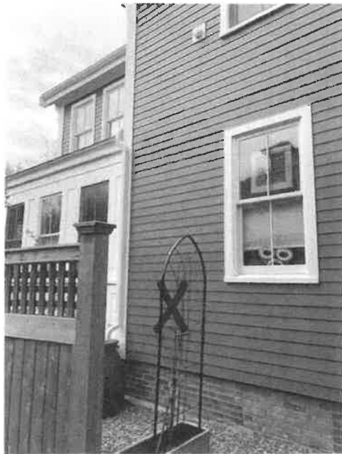
View from east side, showing unit placement.
