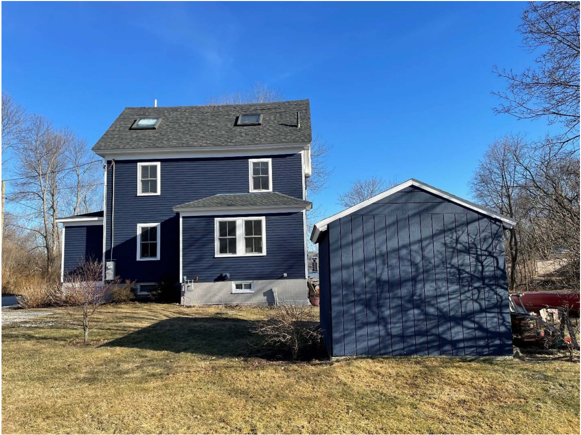
Side View of House & Shed (facing east)
