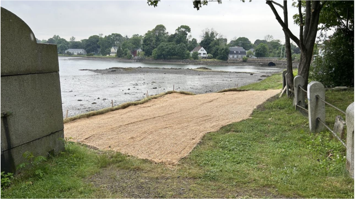
Photo 4 Disturbed area erosion control matting over City wetland buffer seed mix 6-18-24.
