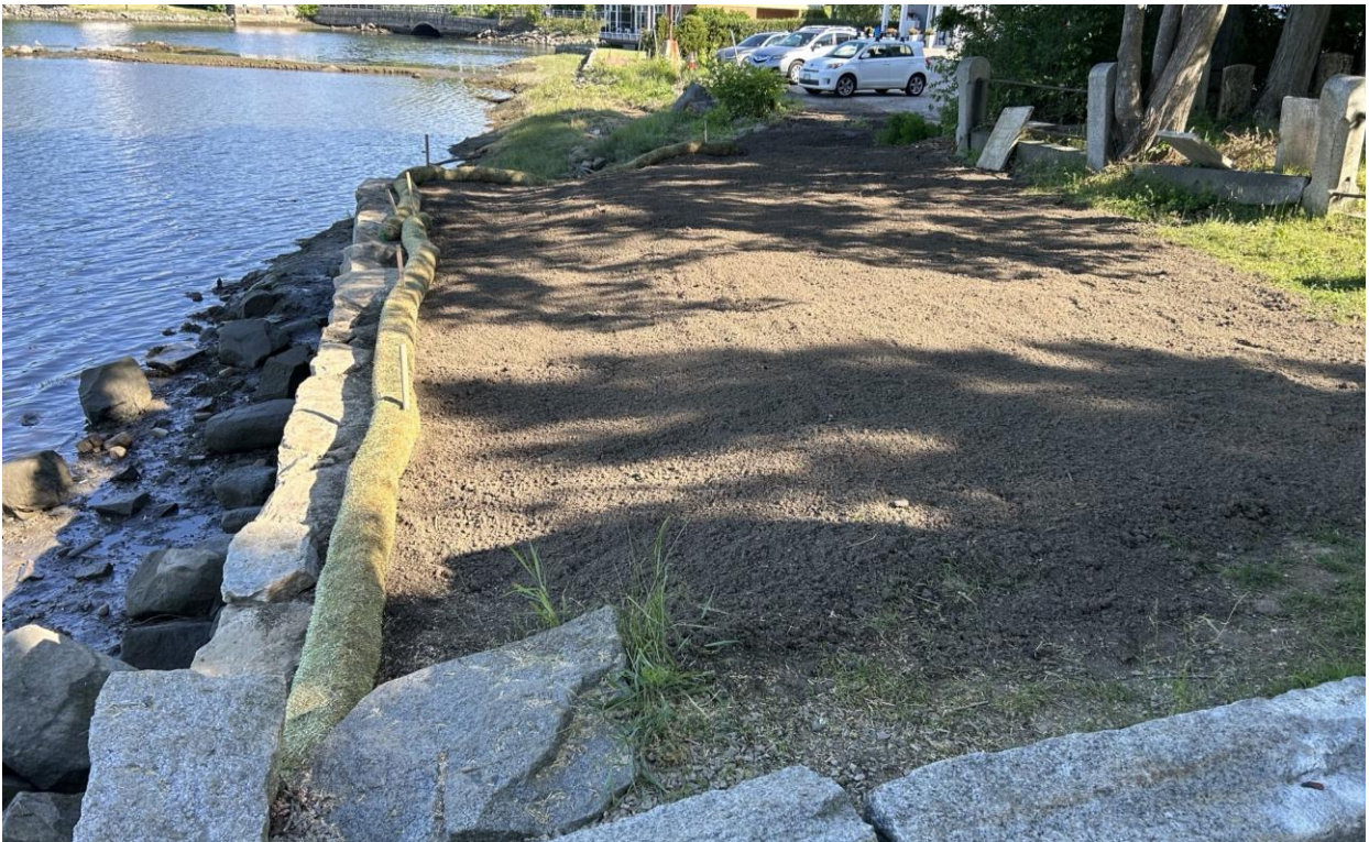
Photo 3 Disturbed area erosion controls and seeding 6-18-24
