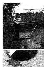
4. Collected rinse water is typically removed by vacuum hose. 5. Reassemble cartridges as detailed later in this document. Reuse
