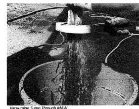
Pressure wash cartridge deck and receptacles to remove all sediment and debris. Sediment should be rinsed into the sump area. Take care not to flush rinse water into the outlet pipe.
