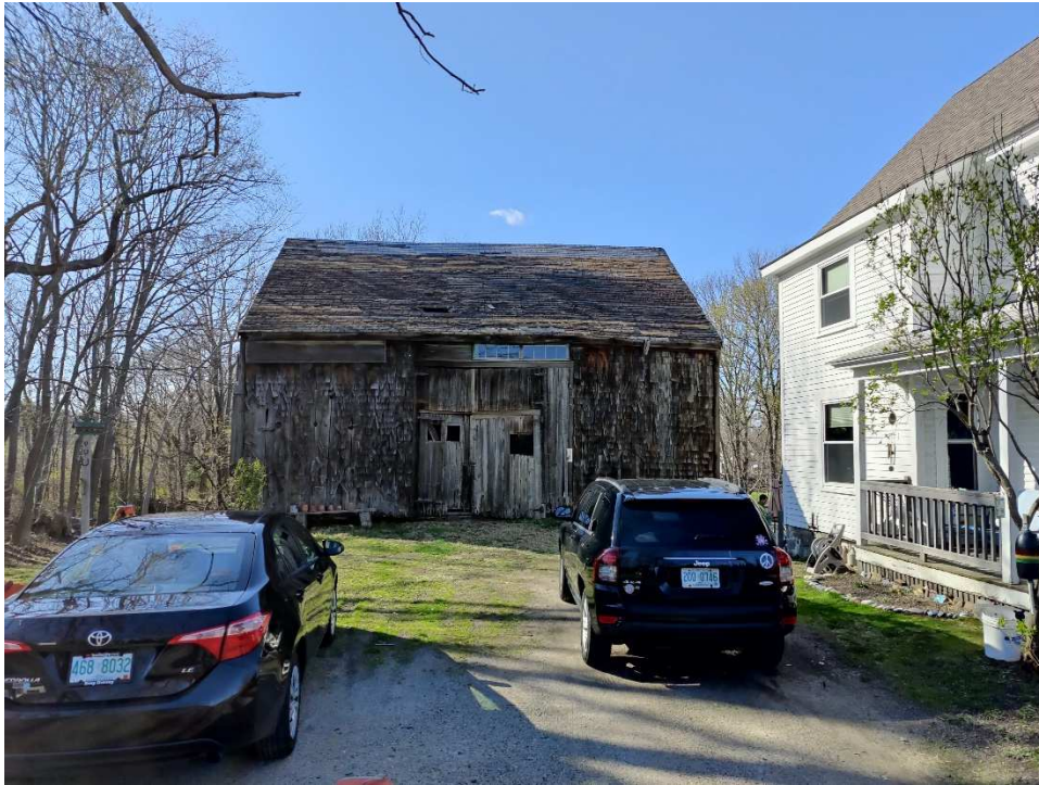
View of barn looking to the north
