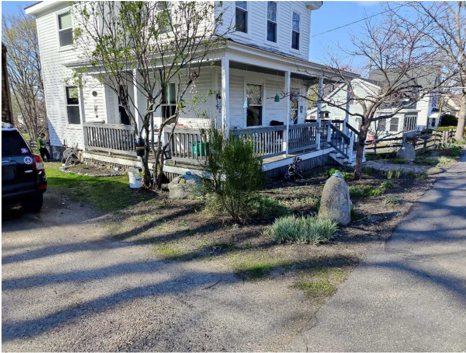
View of house looking to the north
