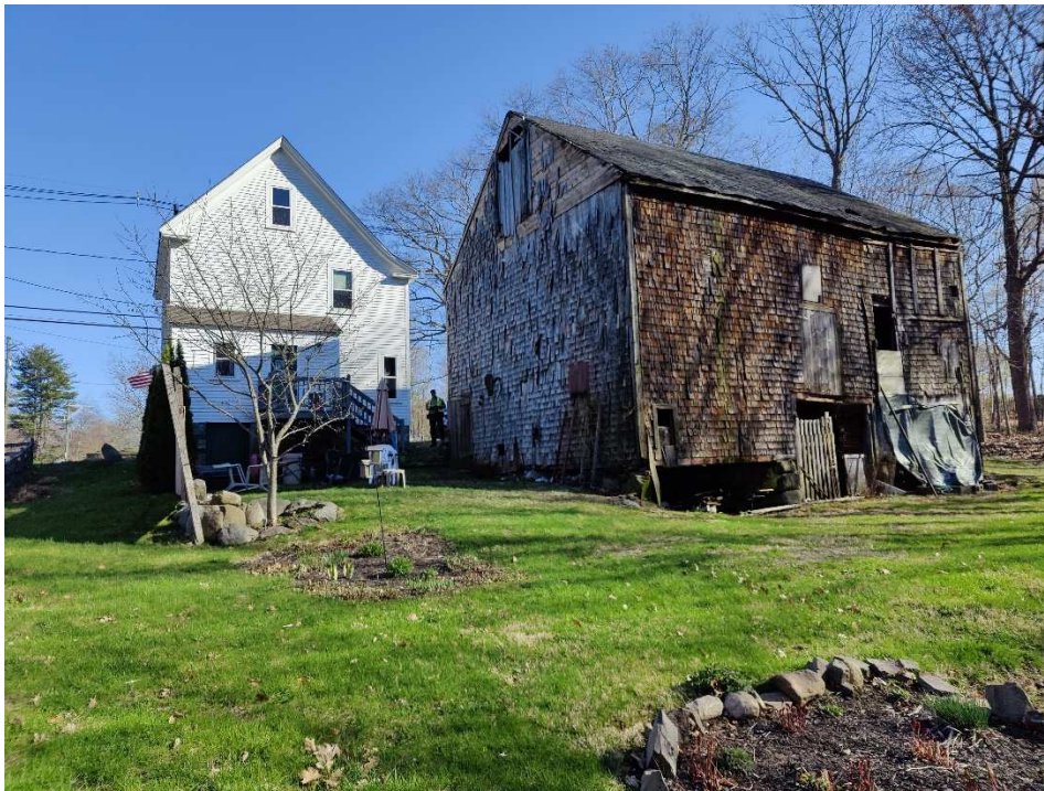
View of barn and house looking to the south
