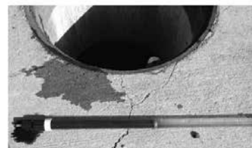
Inspection Utilizing Sediment Probe
