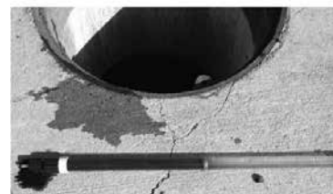
Inspection Utilizing Sediment Probe
