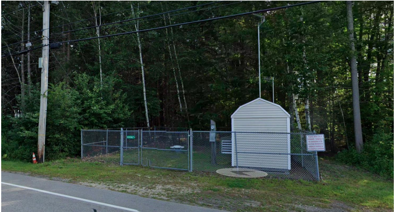
Photograph 3: Existing Pump Station (Facing South)
