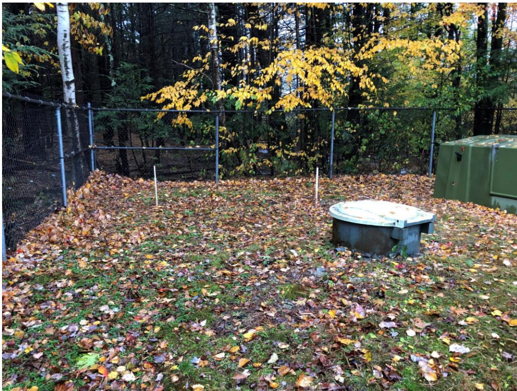
Photograph 2: Existing Pump Station (Facing West)
