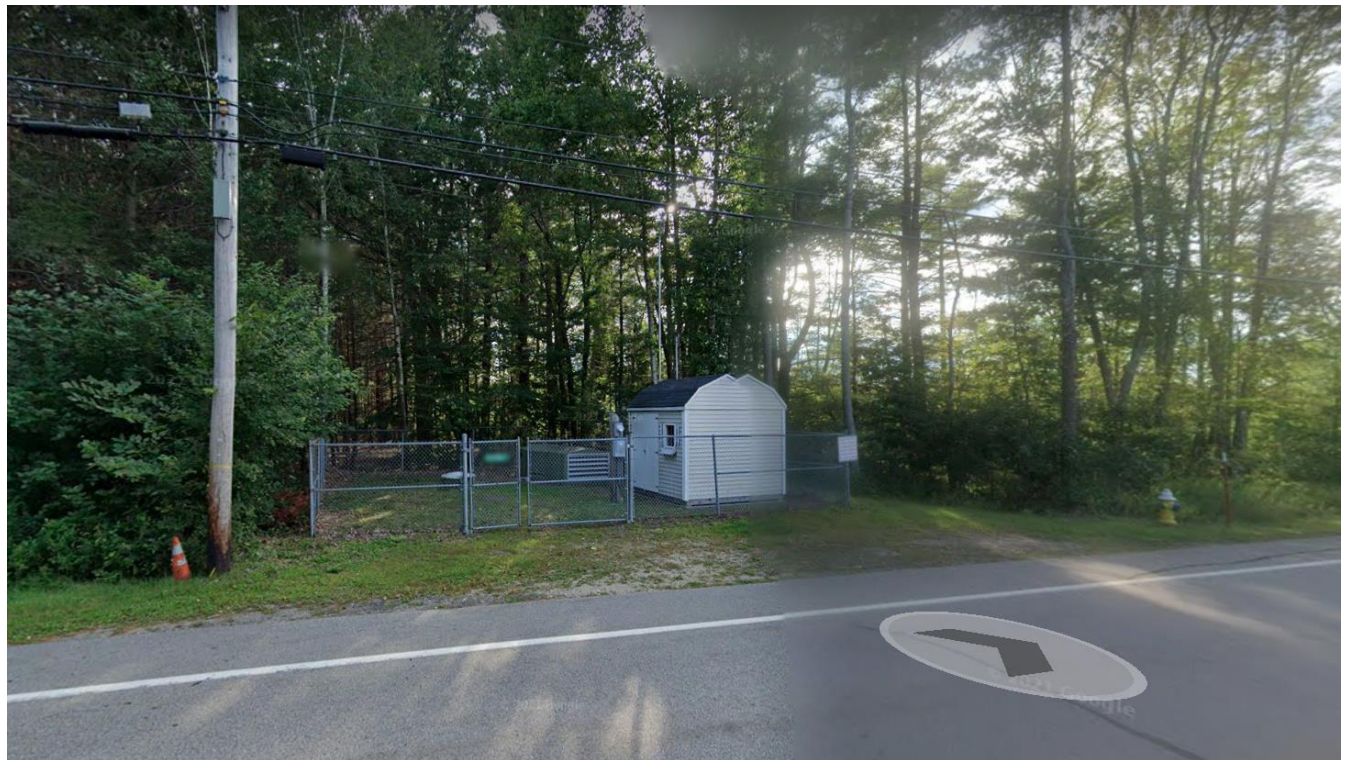
Photograph 4: Existing Pump Station (Facing Southwest)
