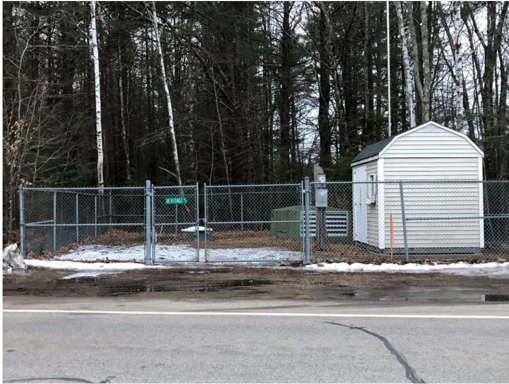
Photograph 1: Existing Pump Station (Facing Southwest)
