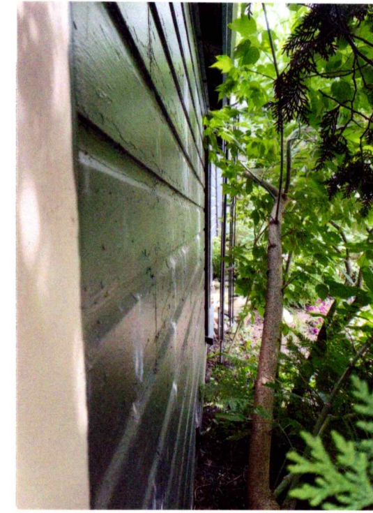
GARAGE EXIST RIGHT SIDE
