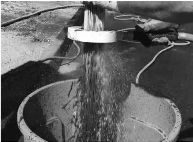
Rinsing Cartridge with Contech Rinse Tool
