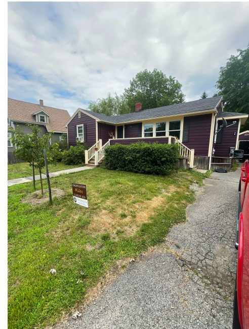
Right side of front yard.
