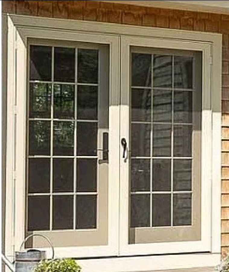
EXISTING 15-LITE FRENCH DOOR PROPOSED 15 LITE DOOR TO MATCH IN PRIMARY PROPOSED TRANSOM INSTALLED OVER THIS RELOCATED 15-LITE DOOR
