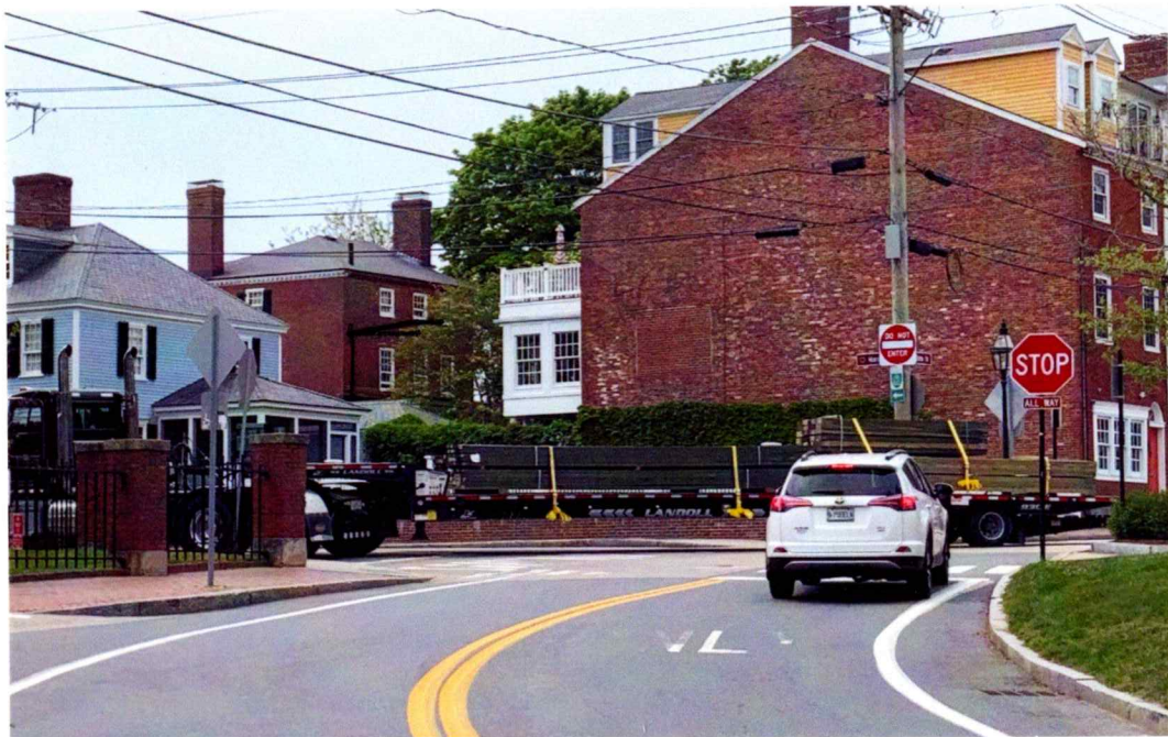
VIEW OF REAR ELEVATION FROM THE CORNER OF MARCY & STATE ST
