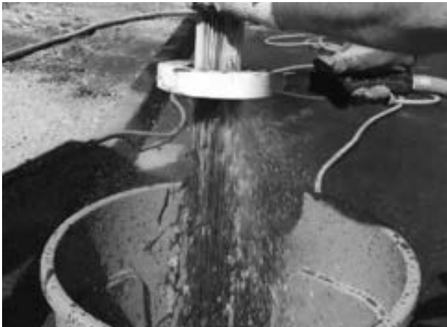
Vacuuming Sump Through MAW
