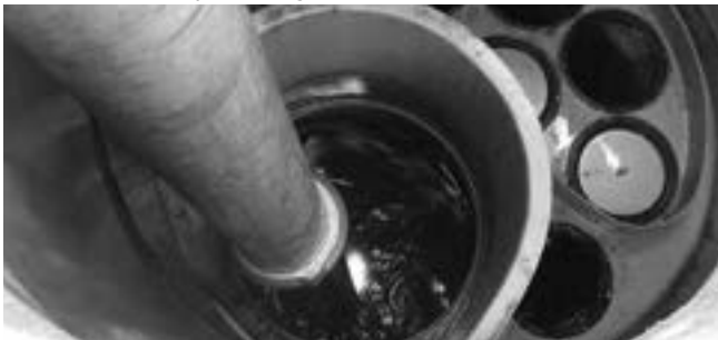
Vacuuming Sump Through MAW
