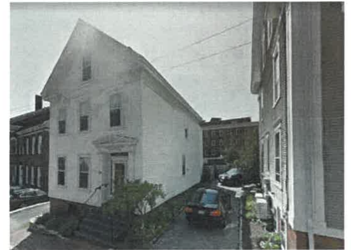
MATERIAL RELATE TO ADJ. STRUCTURE
