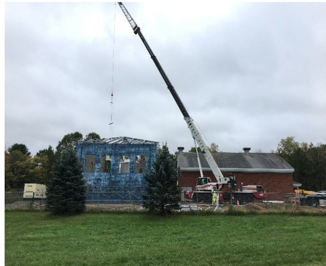
New Building Under Construction
