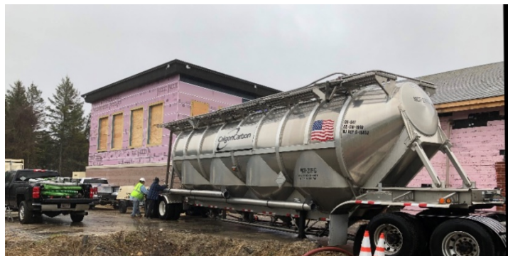
Delivery of Activated Carbon for New Carbon Filters April 2020
