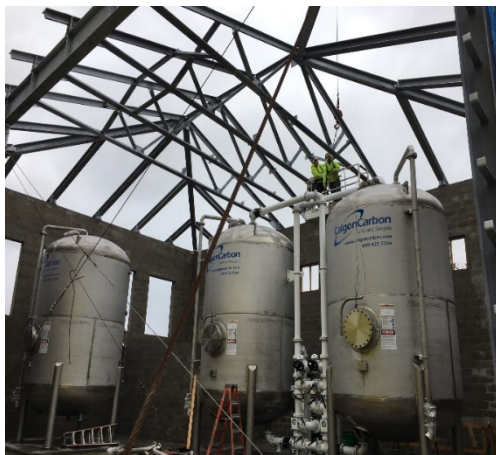
Installation of New Carbon Filters
