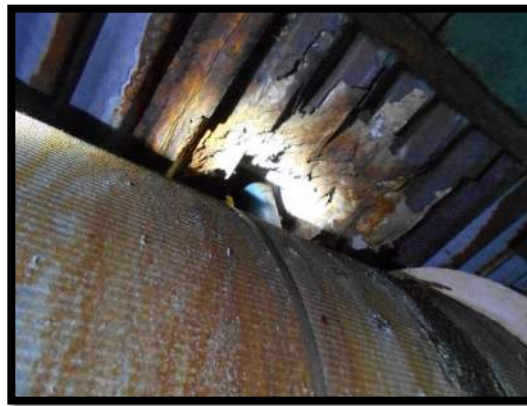
Deck Spall at Northern Air Release Valve
