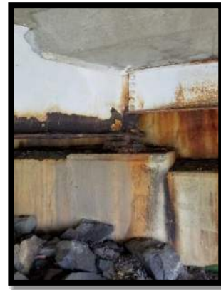
Beam End Deterioration
