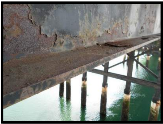
Typical Beam Corrosion
