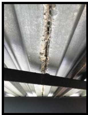
Efflorescence on Underside of Deck
