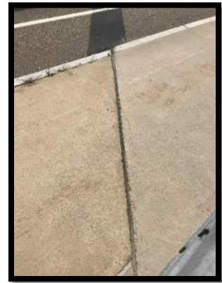
North Sidewalk Expansion Joint
