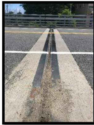
Debris in South Expansion Joint
