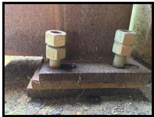
Typical Bent Anchor Bolt
