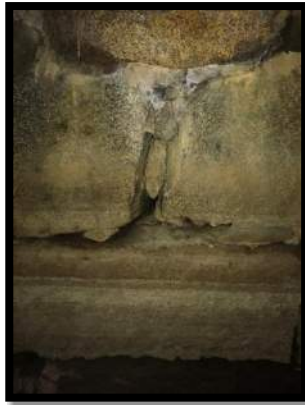
Voids Between Granite Blocks of Abutment
