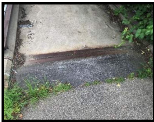
South Abutment Expansion Joint
