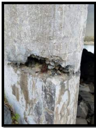
Spall on Southwest Wingwall
