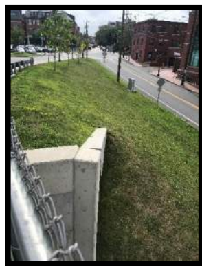
Rotated Southwest Wingwall Coping
