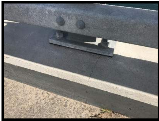
Hairline Crack in Brush Curb
