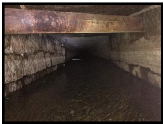
Utility in Hydraulic Opening Near Outlet
