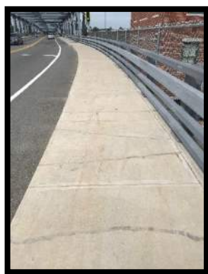
Sidewalk Cracking
