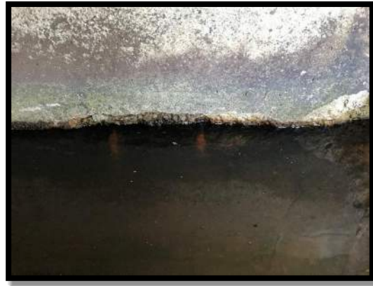
Loss of Concrete Below Waterline
