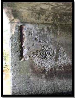
Barrell 2 Abrasion and Exposed Rebar
