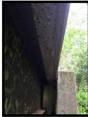
Delamination at Deck Overhang
