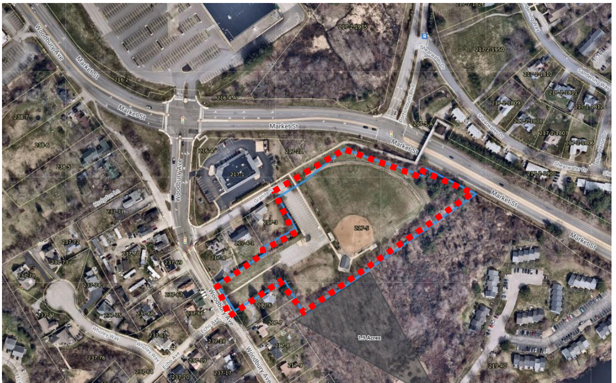
25 Granite Ave. (4A) – Active Recreational Facility
