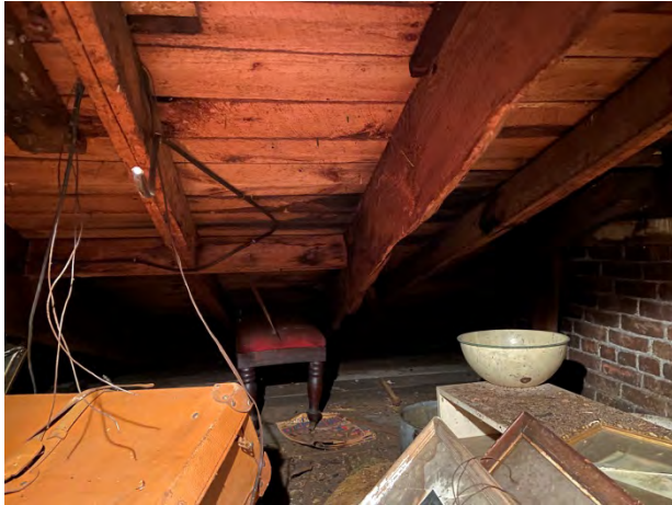
15-Rafters and sheathing above ell
