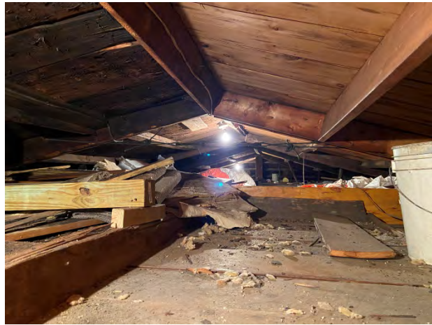
12 - View of repaired roof area
