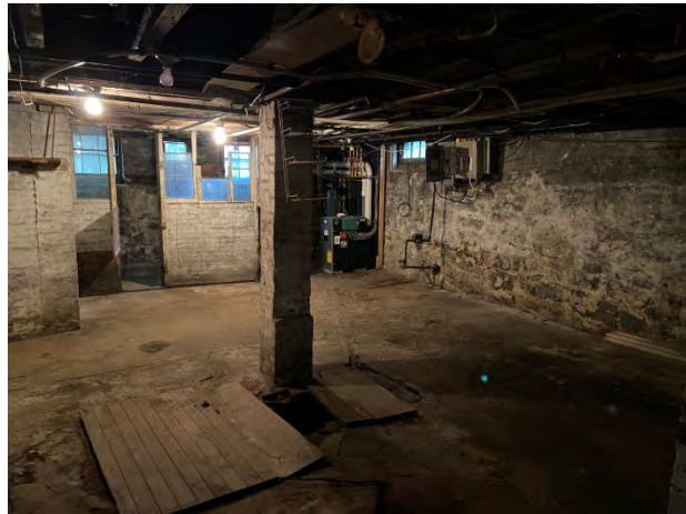
4 – View looking toward front right corner
