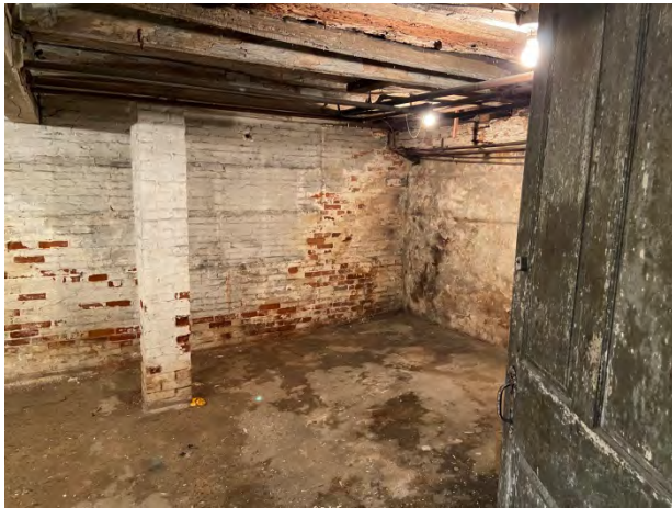
3 - View looking toward front left corner
