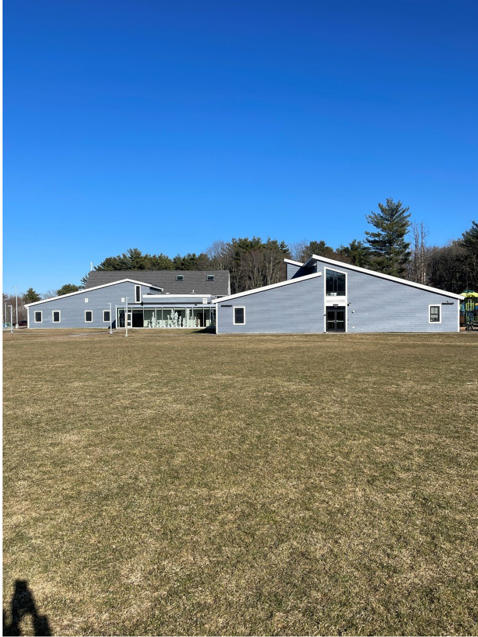
Right Elevation of School Building
