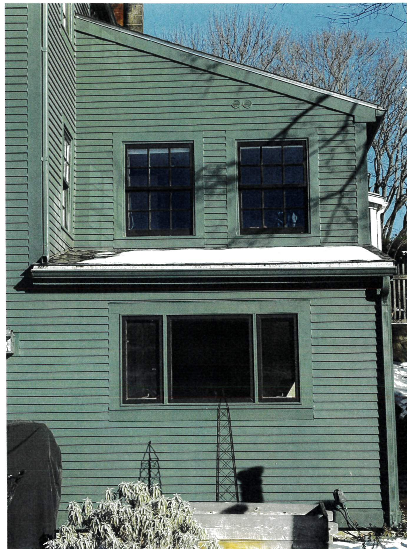
South Elevation: close-up of existing one-story addition
