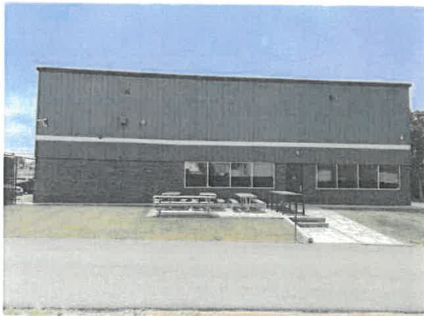
Figure 4: Right side of building, looking south.
