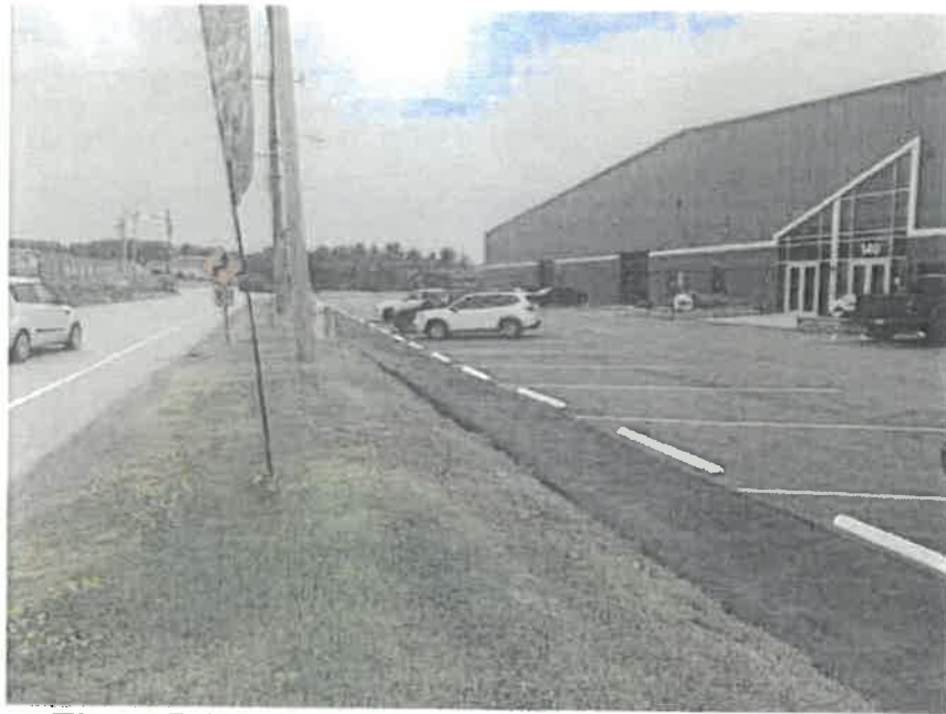
Figure 7: Front parking lot, looking south.
