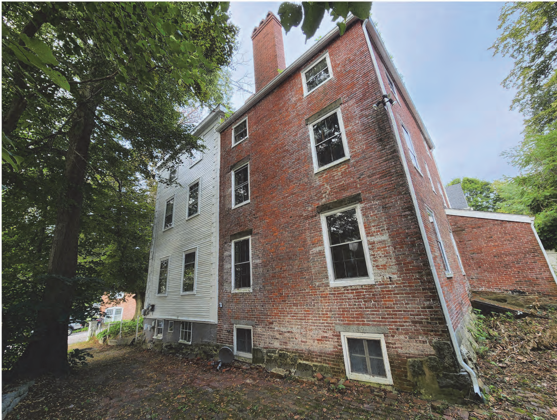
A2.12 EAST EXTERIOR ELEVATION PHOTO EXISTING CONDITIONS
