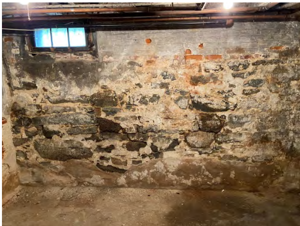
5 - View looking toward front wall
