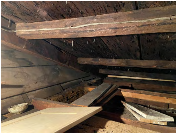
11 - Rafter and purlin framing
