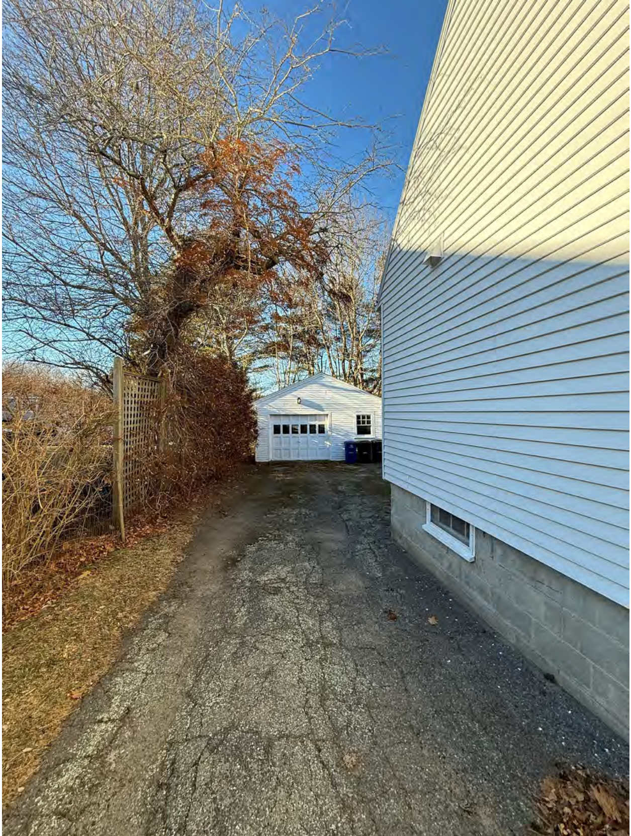
Left Side Toward Existing Garage
