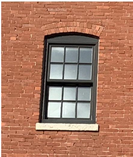
Exterior image of existing window (above)
