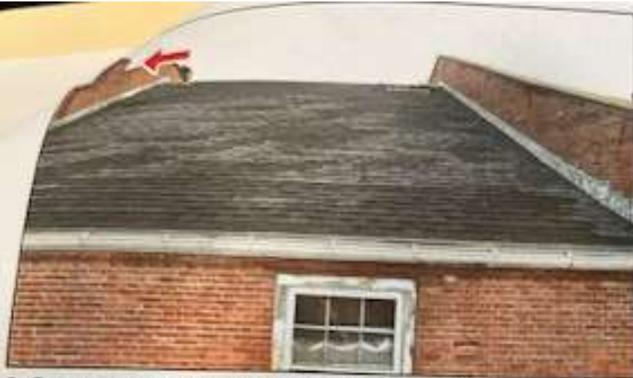
1.0 Item 21(Picture) falling parapet wall
