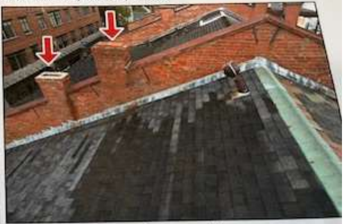
1.0 Item 24(Picture) open chimneys
