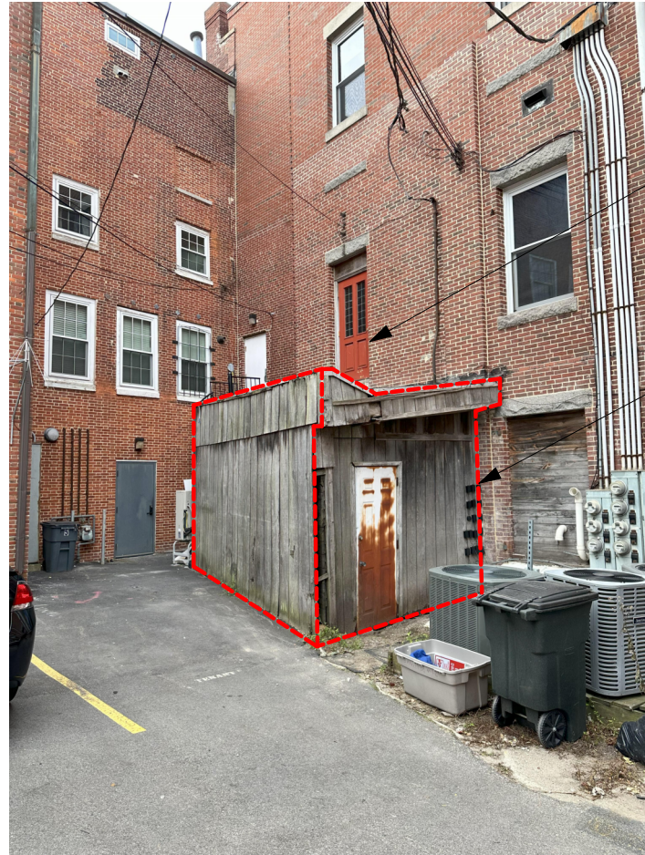
WOOD SHED TO BE REMOVED
