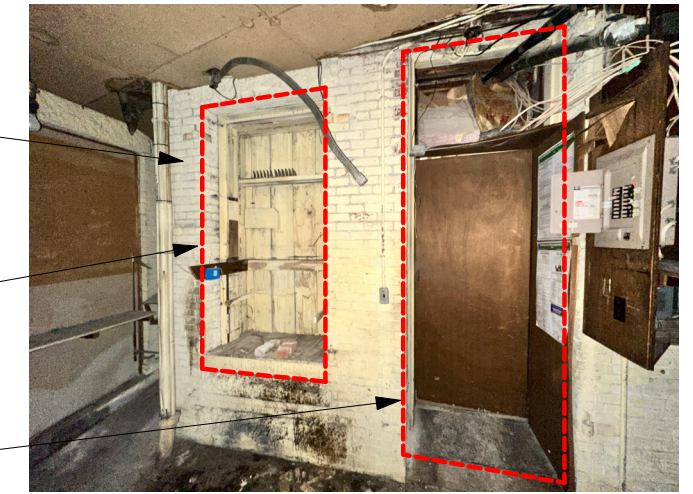
EXTERIOR WALL INSIDE SHED
