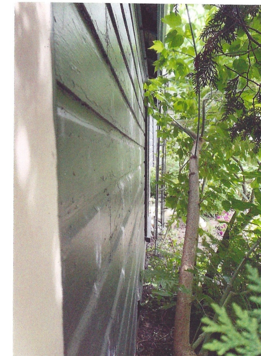
GARAGE EXIST RIGHT SIDE
