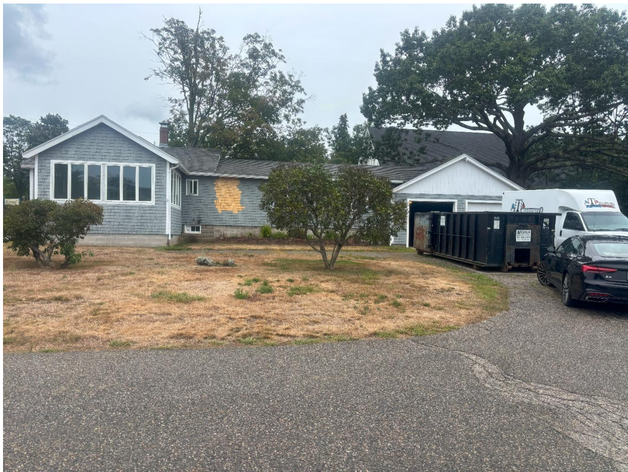
South Elevation of House at 409 Lafayette Road
