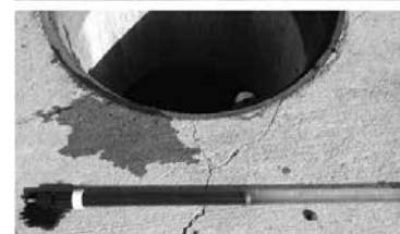
Inspection Utilizing Sediment Probe
