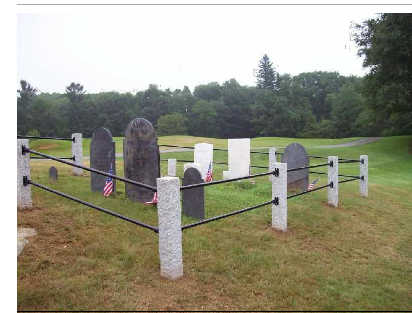
Proposed Memorial and Cemetery Fence - 8x8 granite posts with 2.5" diameter metal rails.
