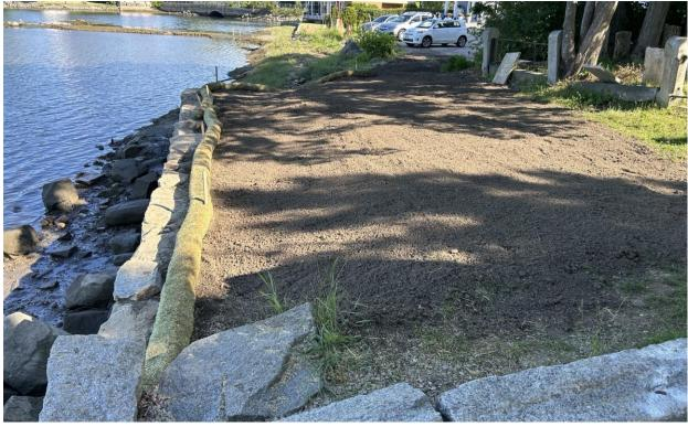
Photo 3 Disturbed area erosion controls and seeding 6-18-24
