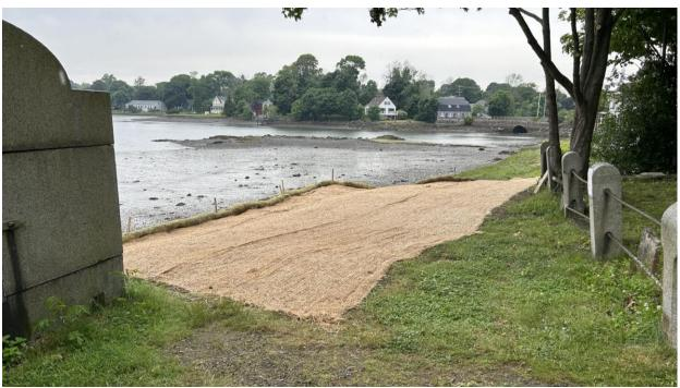
**Photo 4** Disturbed area erosion control matting over City wetland buffer seed mix 6-18-24.
