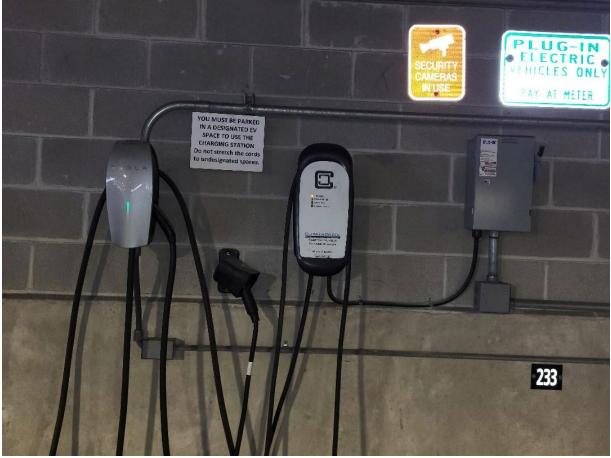
Dover Level 2 Charging Station in Parking Garage. Transformers are behind the wall with all other transformers for the garage and Police Station. No noise could be heard from the station (no one was charging at the time). The Parking Dept shared, they have received no complaints regarding the charging station in the garage. It is on the second floor, about 100' or more from senior housing and a restaurant on the other side of the garage.
