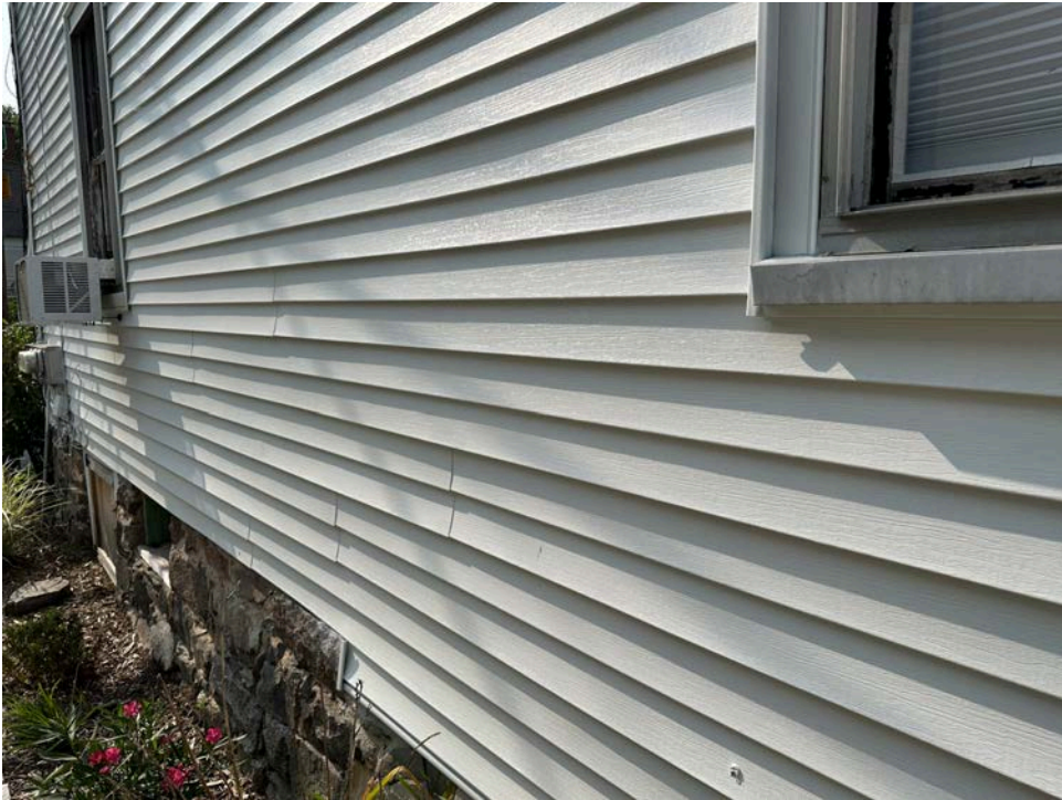
Image #21. VINYL SIDING RIGHT ELEVATION
