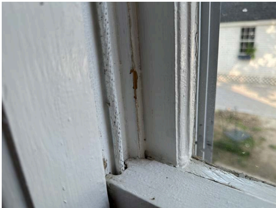
Image #48. PAINTED ROPE AND WEIGHT MECHANISM REAR ELEVATION
