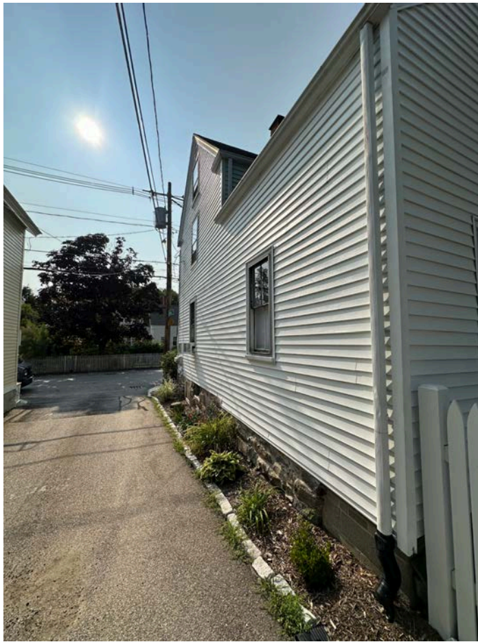
Image #5. EXISTING RIGHT ELEVATION VIEW DOWN HOLMES COURT TOWARD MARCY STREET
