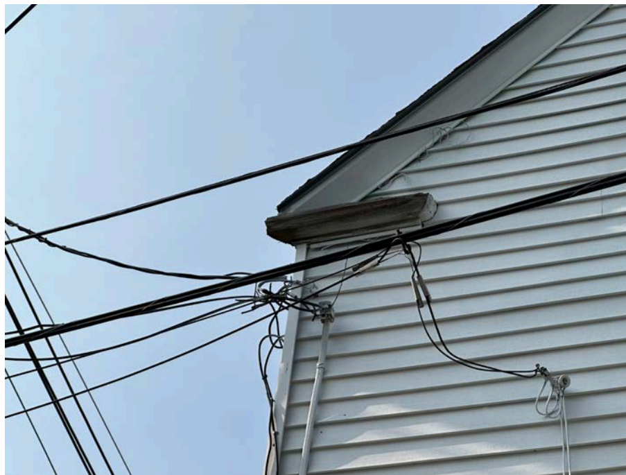
Image #16. CORNICE RETURN AT HOLMES COURT RIGHT ELEVATION
