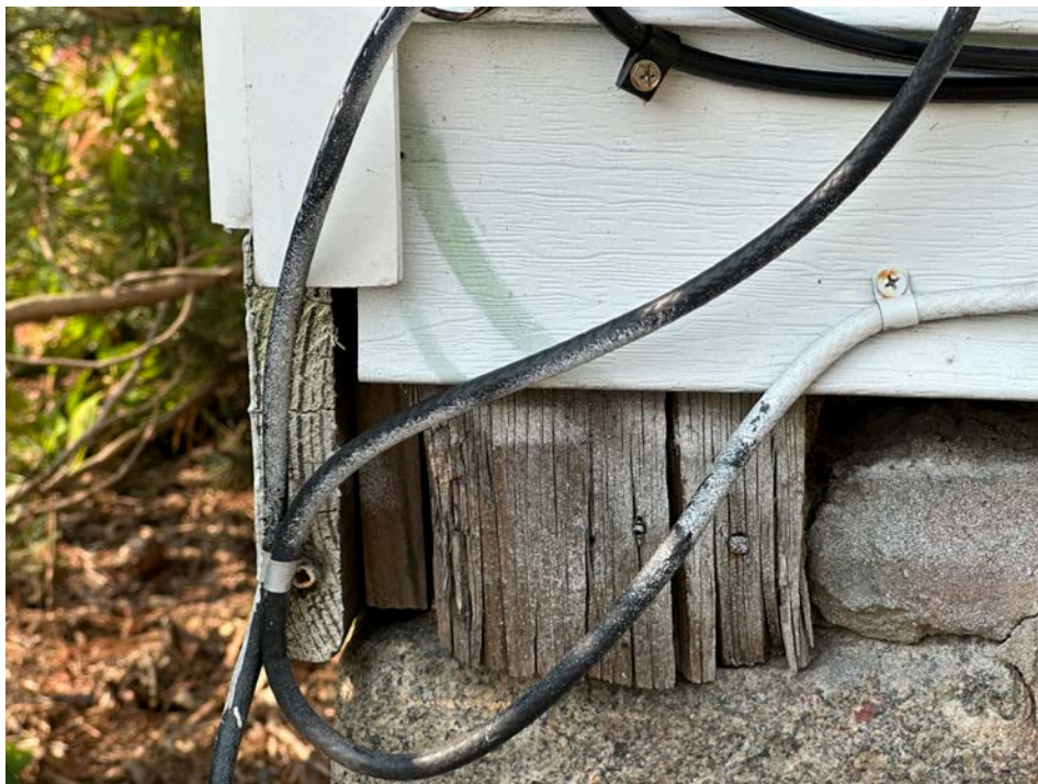
Image #32. EXPOSED STRUCTURAL BEAM CORNER OF MARCY STREET AND HOLMES COURT
