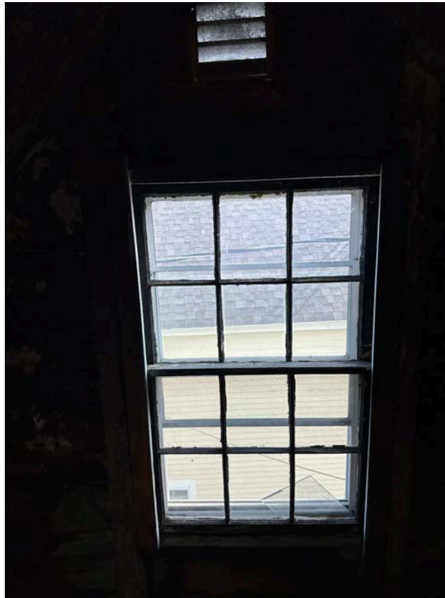
Image #64. ATTIC WINDOW RIGHT ELEVATION
