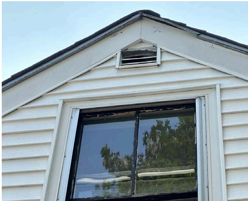
Image #29. ROOF LINE REAR ELEVATION, LEFT SIDE
