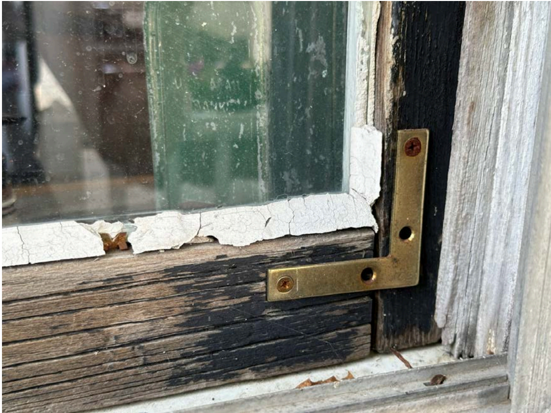
Image #45. REPAIR TO WINDOW FRAME REAR ELEVATION, RIGHT
