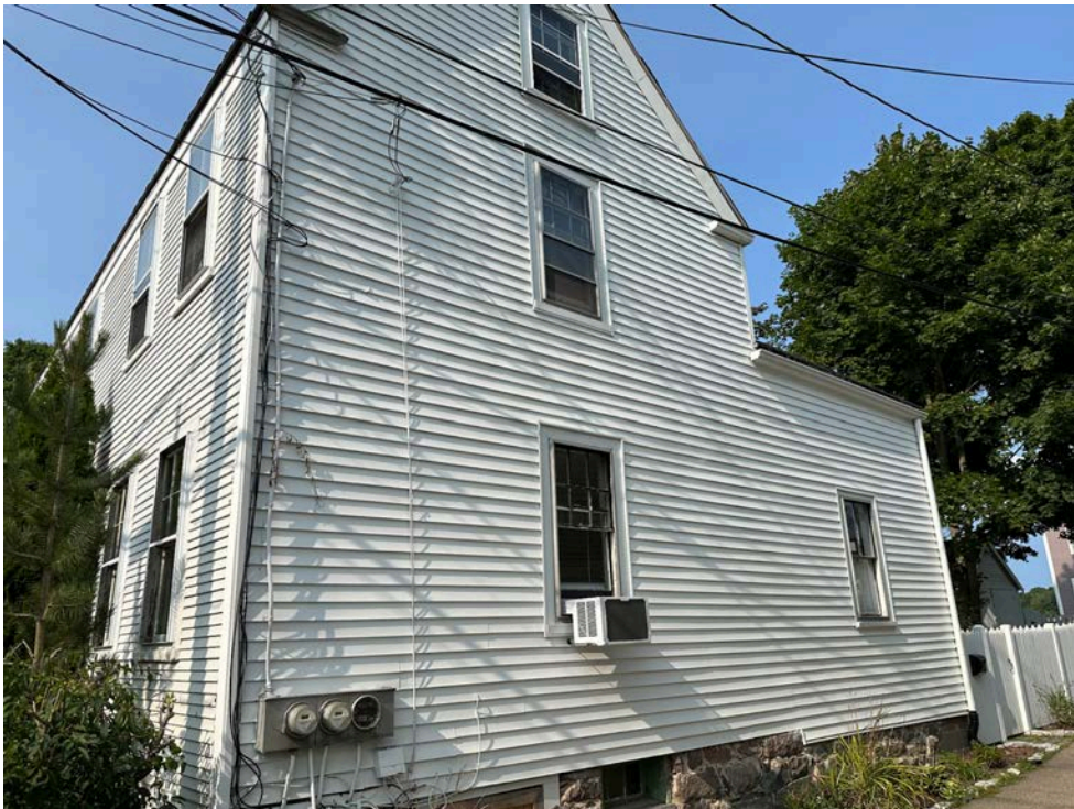
Image #4. EXISTING RIGHT ELEVATION VIEW FROM INTERSECTION OF MARCY STREET & HOLMES COURT
