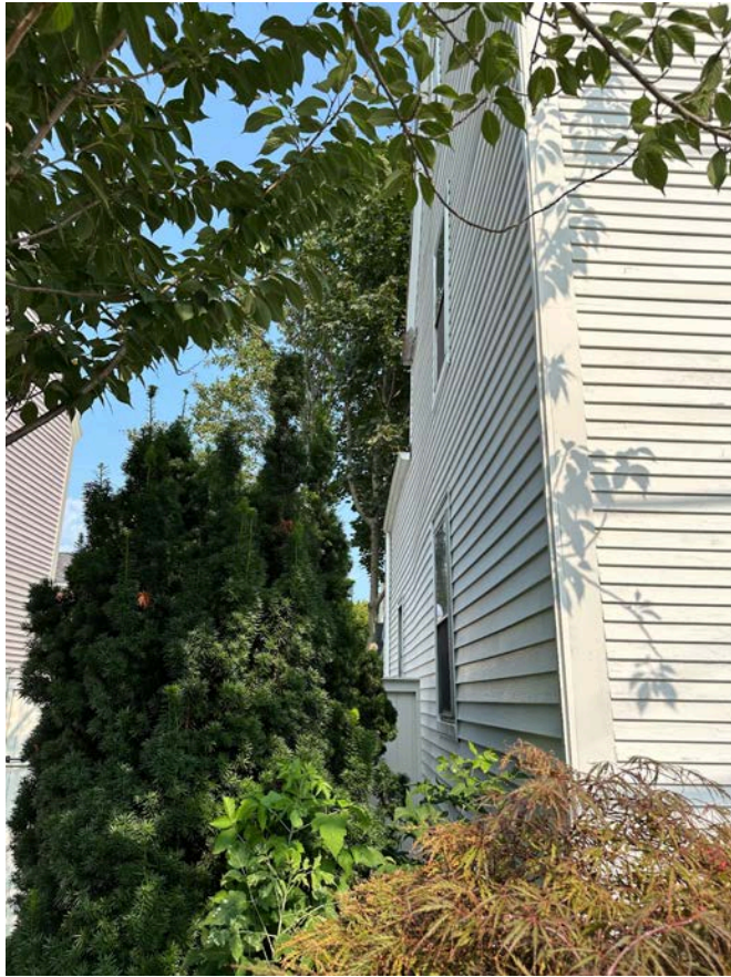
Image #3. EXISTING LEFT ELEVATION VIEW FROM MARCY STREET
