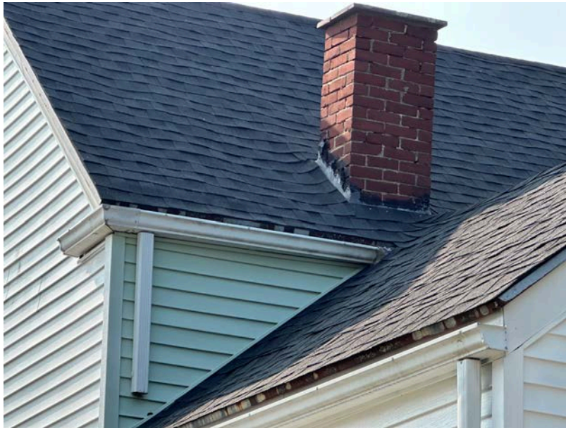
Image #27. CHIMNEY REAR ELEVATION, LEFT SIDE
