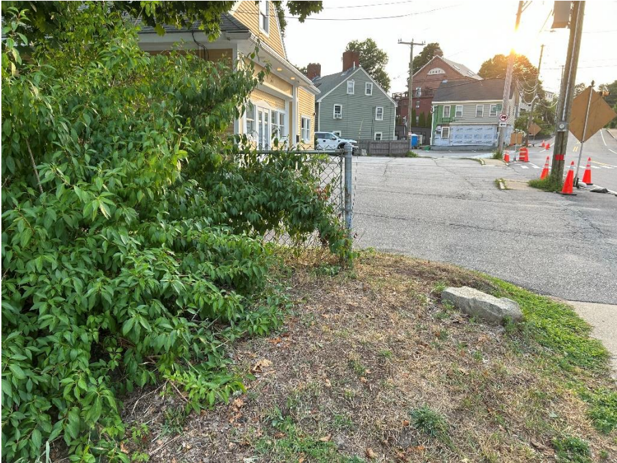
Sample of existing chain link fence to be replaced:
