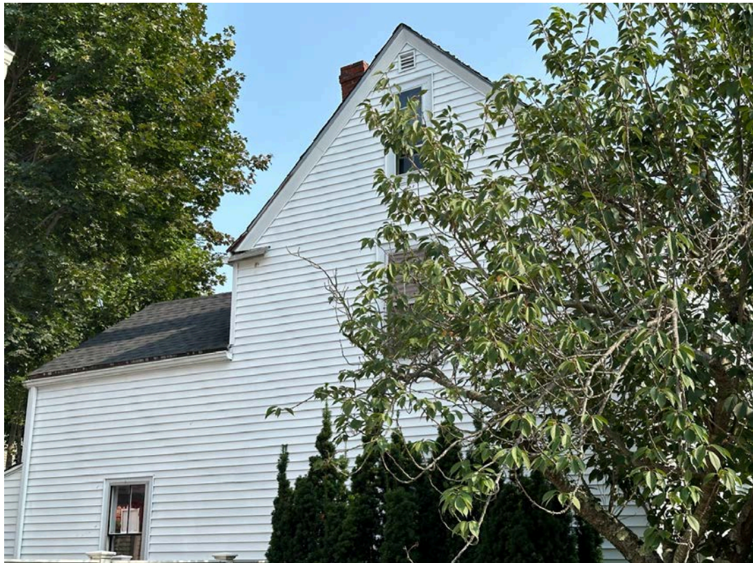
Image #2. EXISTING LEFT ELEVATION VIEW FROM MARCY STREET
