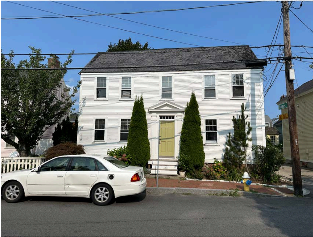
Image #1. EXISTING FRONT ELEVATION VIEW FROM MARCY STREET
