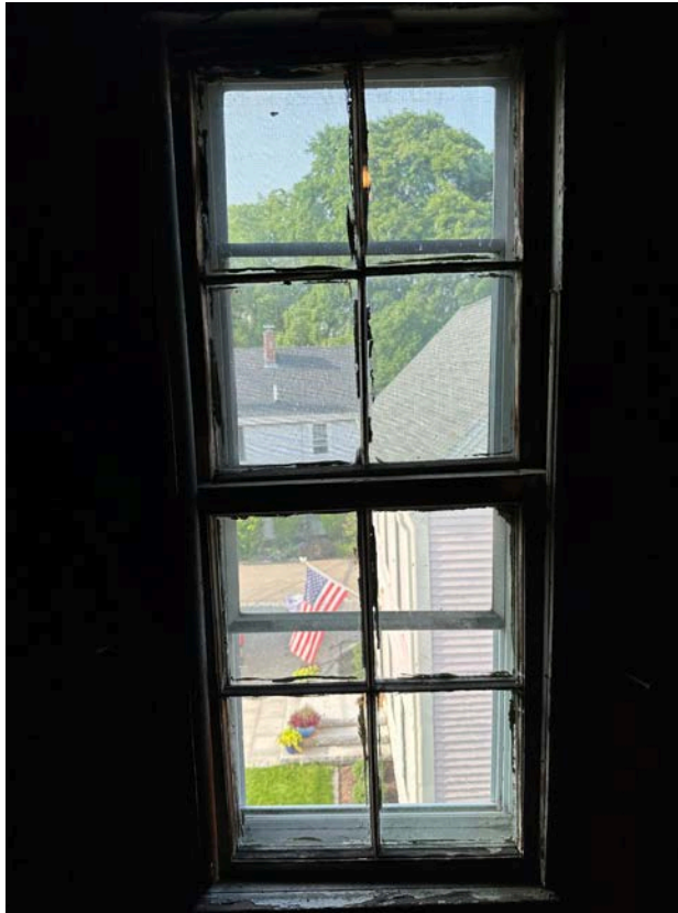
Image #61. ATTIC WINDOW, FROM INTERIOR LEFT ELEVATION
