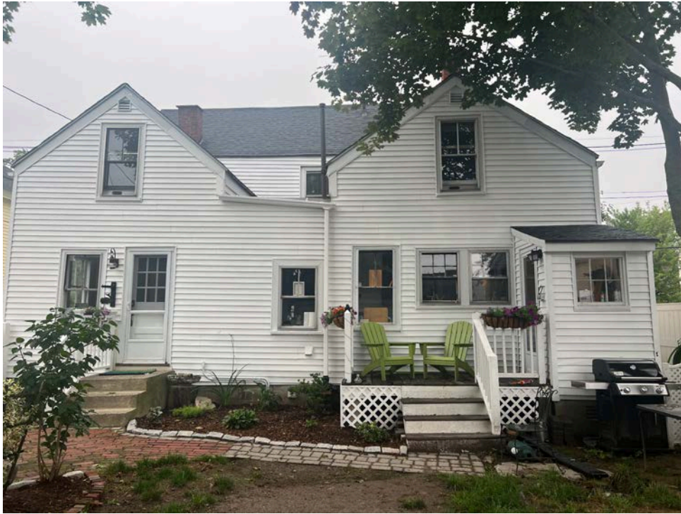
Image #7. EXISTING REAR ELEVATION VIEW FROM BACK YARD
