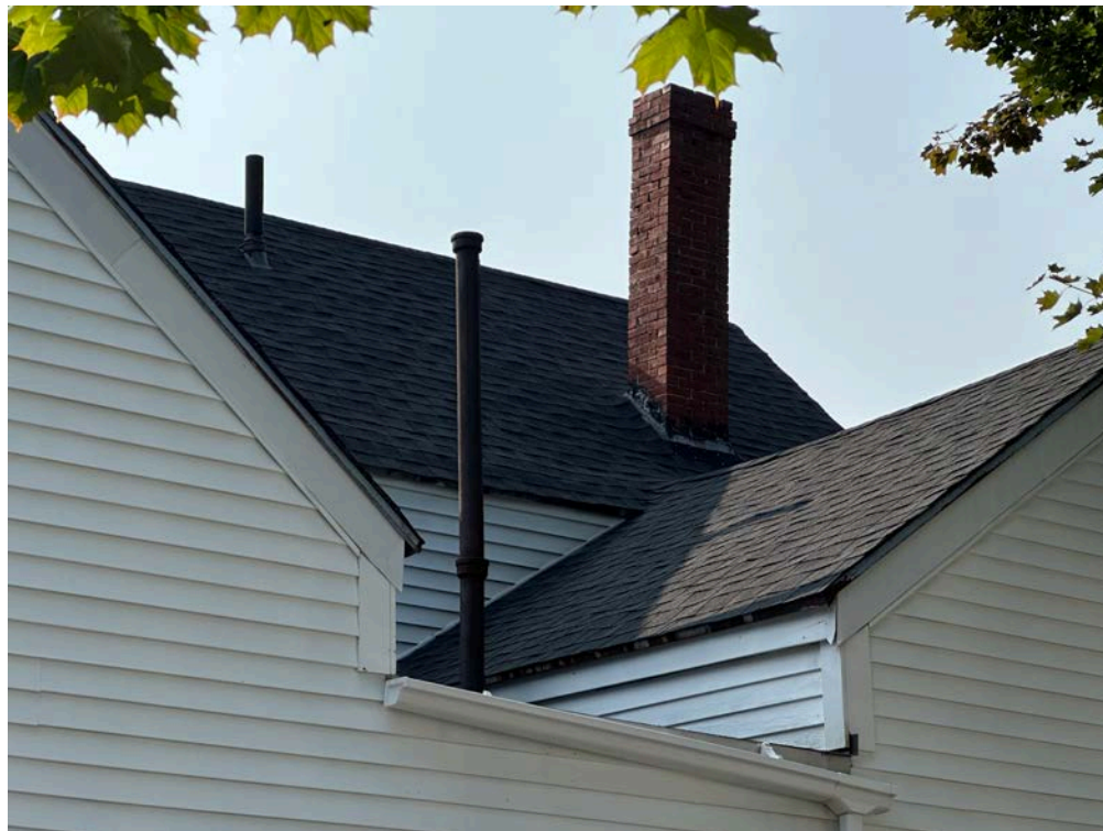
Image #28. CHIMNEY AND VENTS REAR ELEVATION, RIGHT SIDE
