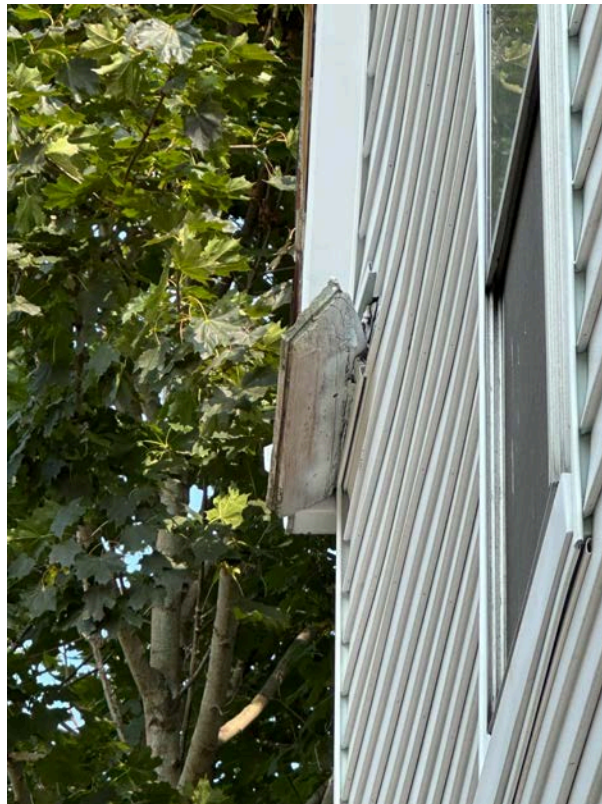
Image #17. CORNICE RETURN AT REAR LEFT REAR ELEVATION
