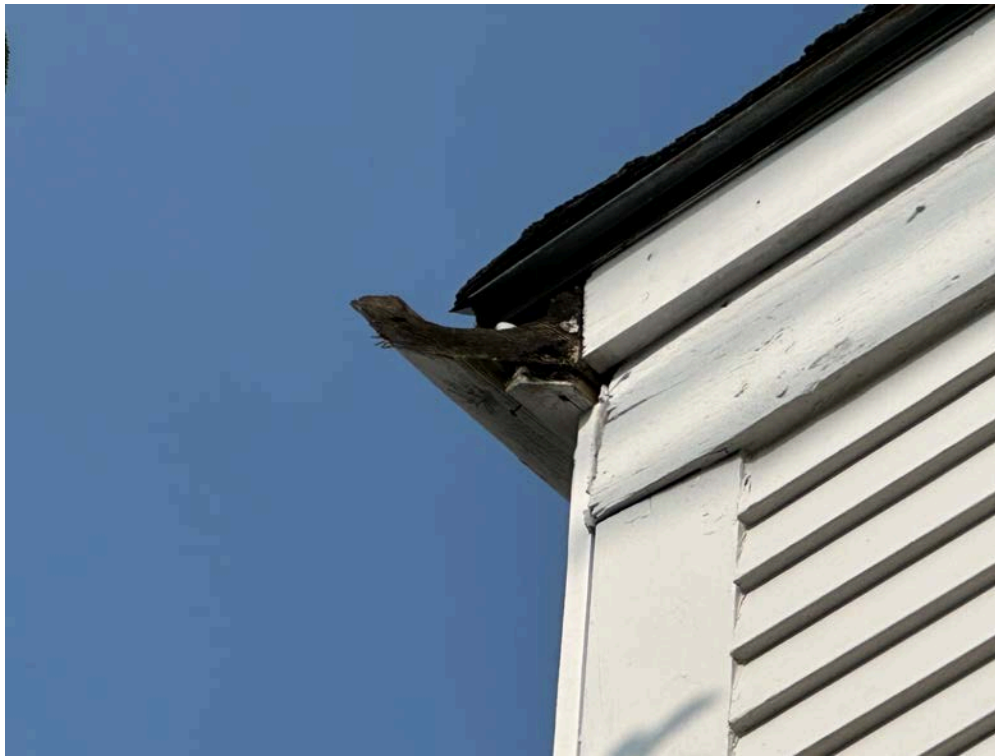
Image #15. CORNICE RETURN AT MARCY STREET FRONT ELEVATION
