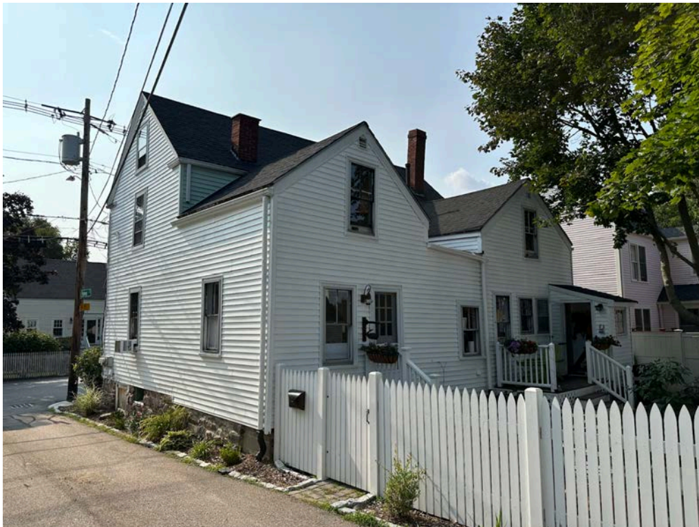
Image #6. EXISTING RIGHT AND REAR ELEVATIONS VIEW FROM HOLMES COURT, MARCY STREET AT FAR LEFT
