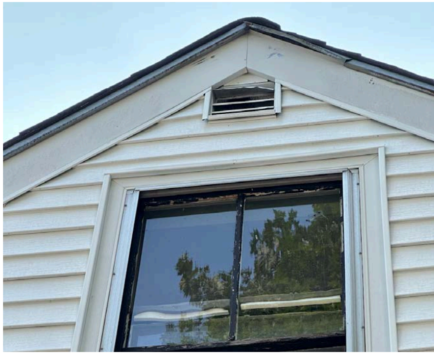
Image #29. ROOF LINE REAR ELEVATION, LEFT SIDE
