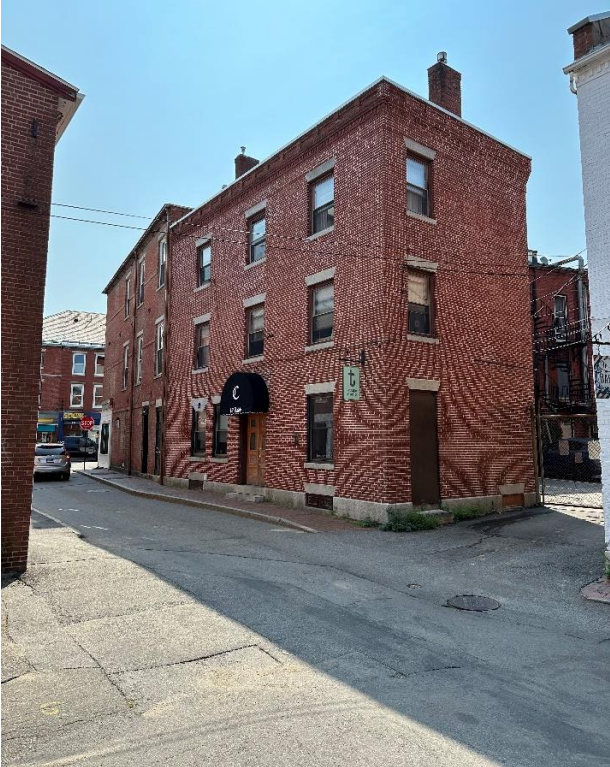
Figure 1 18 Ladd Street from South West
