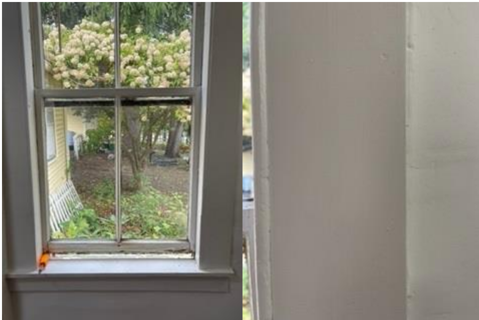
Closeup Restored Interior Frames (all original wood)
