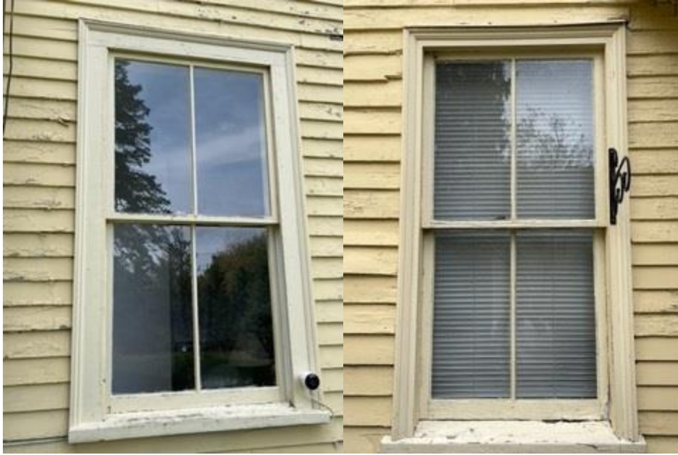
Closeup of Rebuilt Sills and Frames (note where sills were rebuilt at same 14 degree slope)
